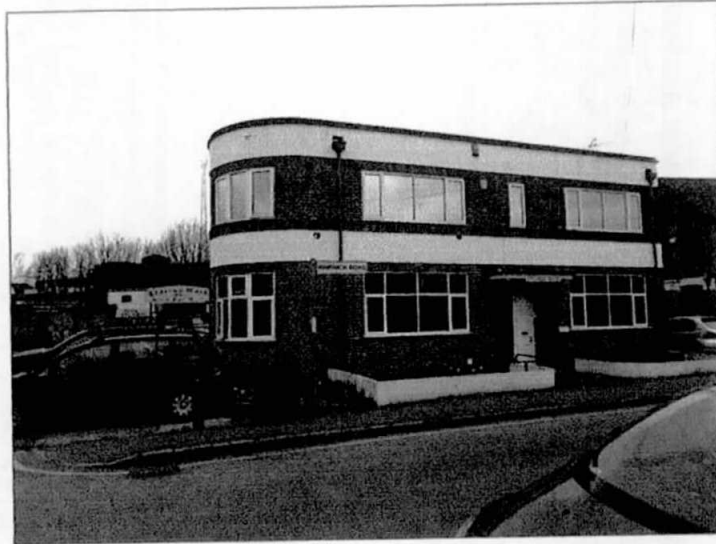
Photograph 1: Office building on the south-west corner of the site, taken from Warwick Road.
