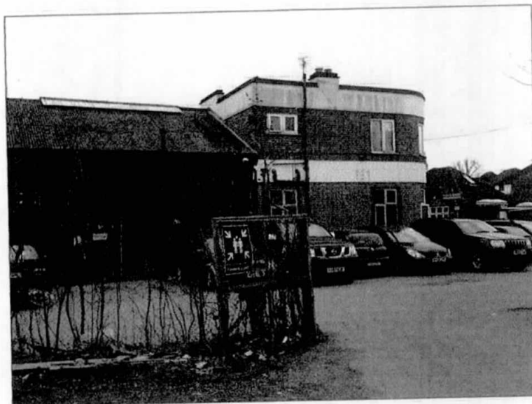
Photograph 4: Suspected asbestos on the roof of the blue units on the left.
