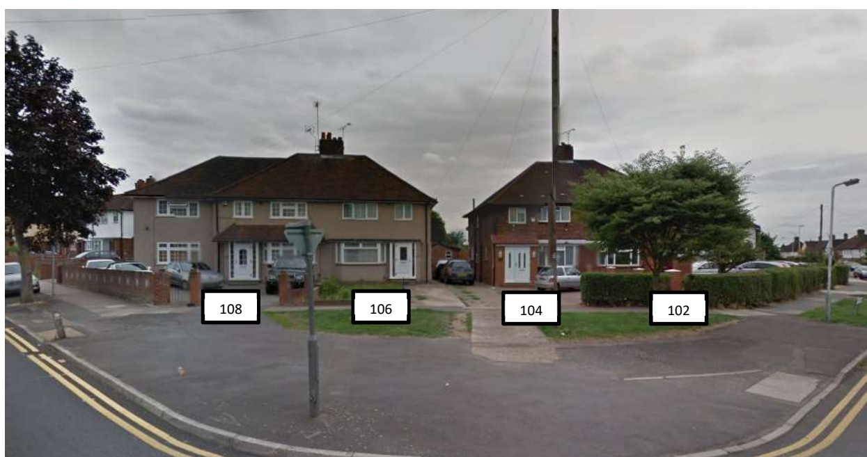
Figure 1 - No.106 and No.108 Apple Tree Avenue
