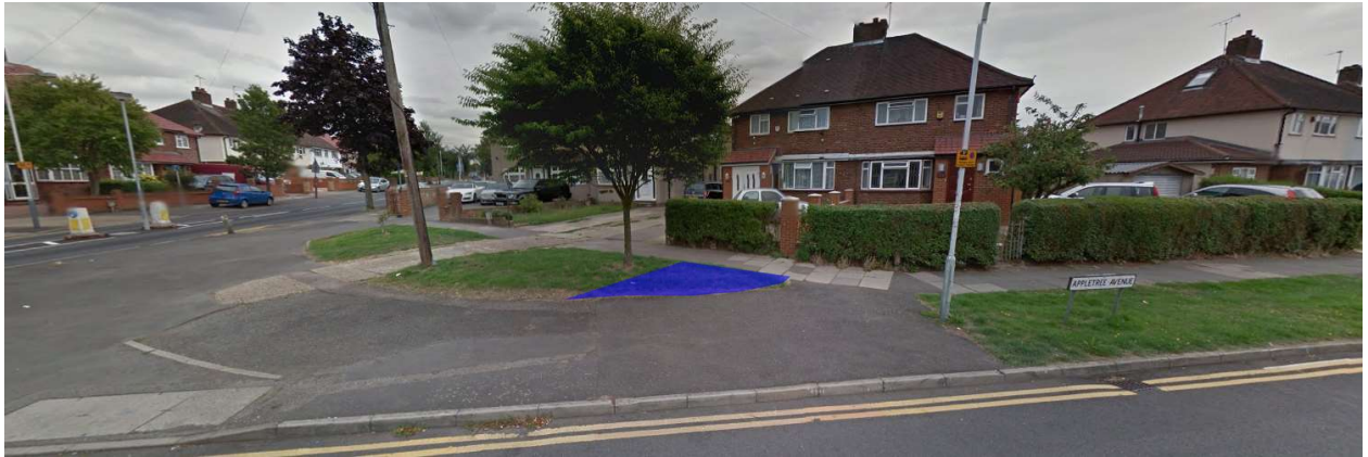
Figure 6 - Grass verge to be removed
