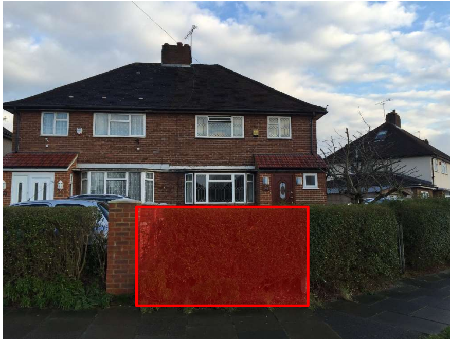
Figure 5 – Hedge area to be removed
