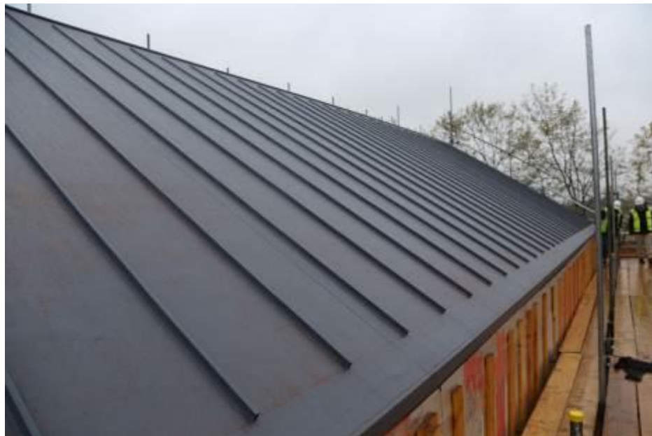
Photo. No. 5 Example of Roof Cladding System.
