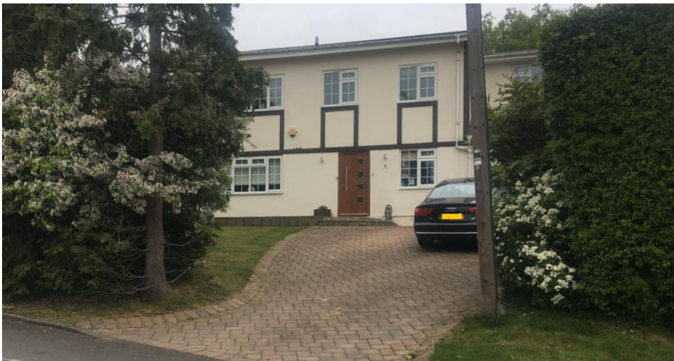
Figure. 5 – No. 31 Weiland Road
