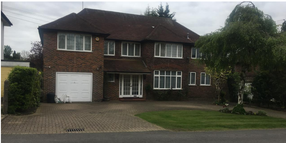
Figure 1 – The application site (front elevation)
