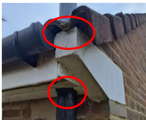
Plate 4.11: Gap in soffit box (north west corner)
