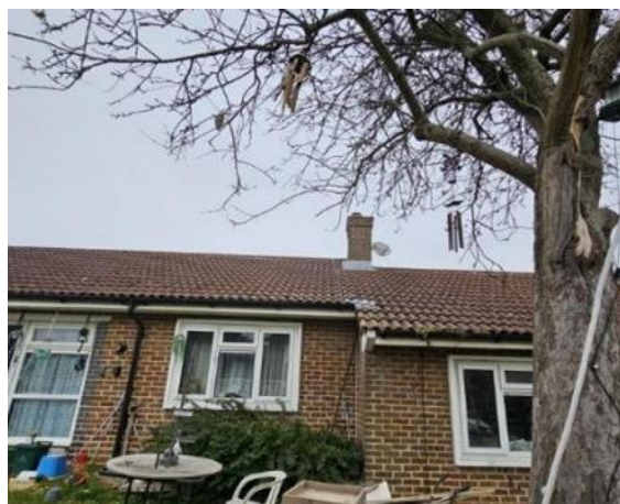
Plate 4.7: Gap in eave tiles (north elevation)
