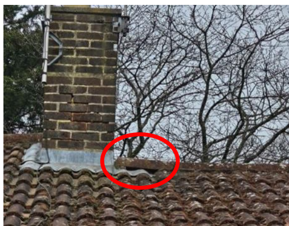
Plate 4.4: Gap in ridge tile
