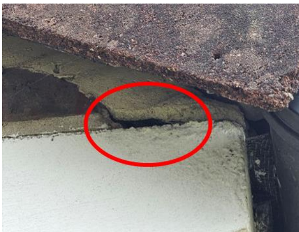
Plate 4.5: Gap in soffit box (south west corner)
