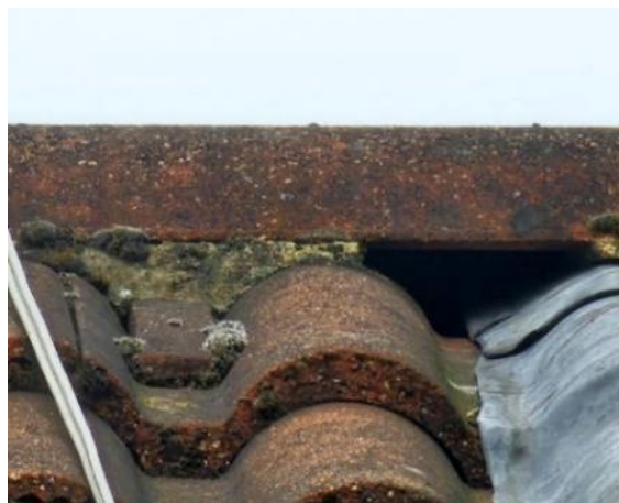
Plate 4.9: Gap in ridge tiles
