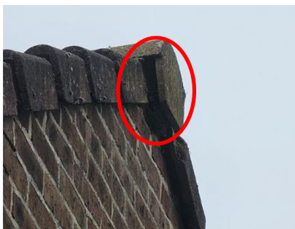
Plate 4.3: Gap in gable end tile (eastern elevation)
