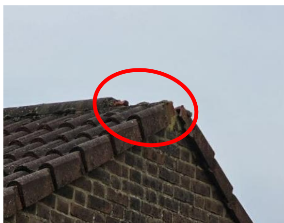
Plate 4.15: Missing ridge tiles (western elevation)
