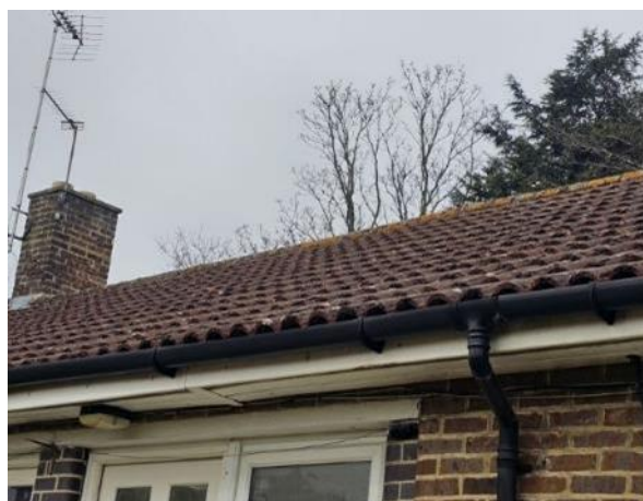
Plate 4.2: Gaps in eave tiles (southern elevation)
