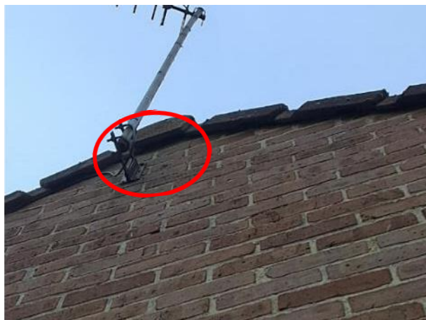
Plate 4.8: Gap in gable end tile (eastern elevation)
