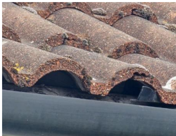
Plate 4.13: Gap in eave tiles (northern elevation)
