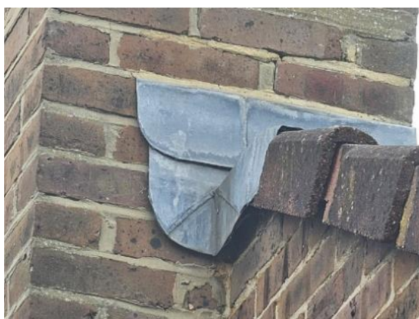
Plate 4.10: Lifted lead flashing (southern elevation)
