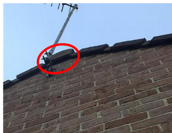
Plate 4.14: Gap in tiles at gable end (eastern elevation)
