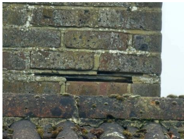
Plate 4.17: Damaged brick work on chimney stack (northern elevation)
