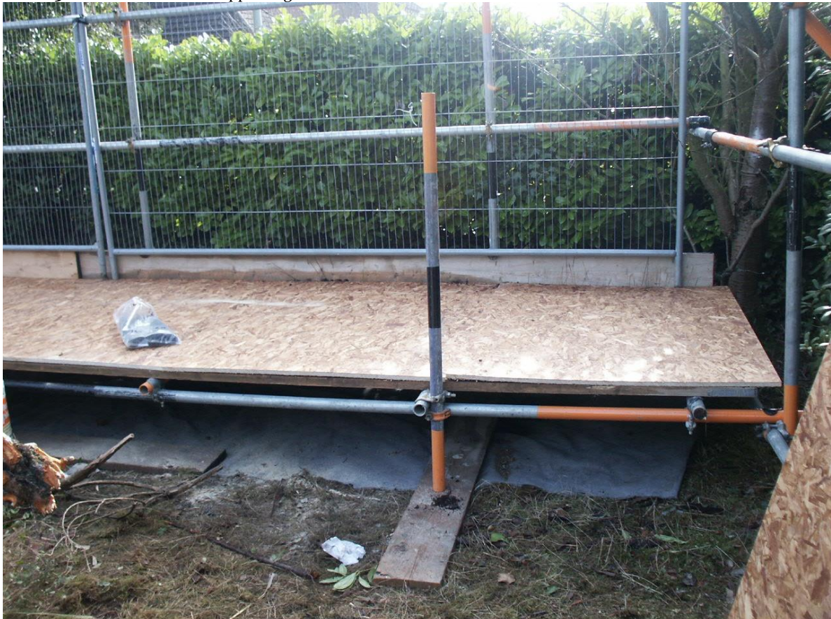
Photo 3 Scaffold framework supporting wooden boards
