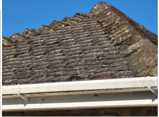
Figure 18. Example of tightly fitted roof and bonnet tiles
