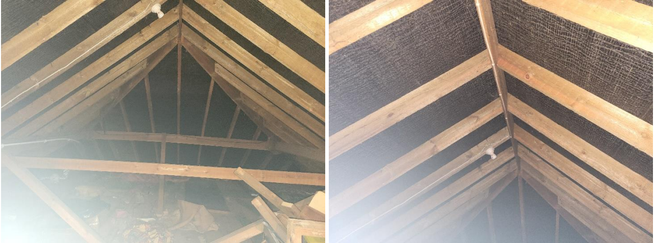
Figure 23. View of the roofing underlay between the rafters and the roof tiles
