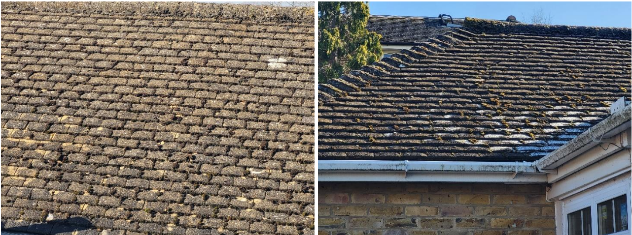
Figure 17. Example of tightly fitted roof and ridge tiles
