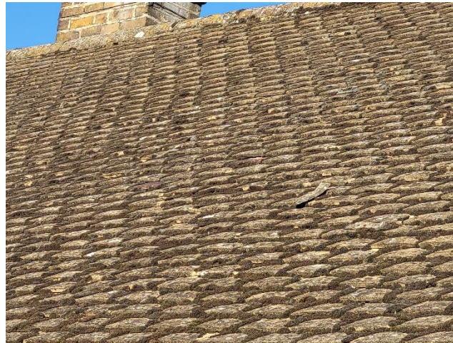
Figure 19. Example of tightly fitted roof and ridge tiles
