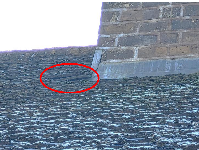
Figure 20. Lifted tiles – front elevation (left) - Lifted tiles – rear elevation (right)
