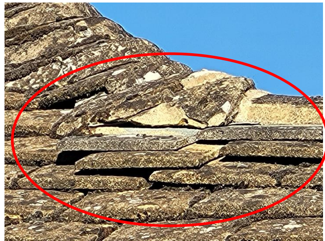
Figure 20. Lifted tiles – front elevation (left) - Lifted tiles – rear elevation (right)
