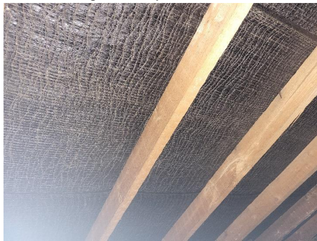
Figure 24. View of the roofing underlay between the rafters and the roof tiles
