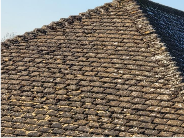
Figure 18. Example of tightly fitted roof and bonnet tiles
