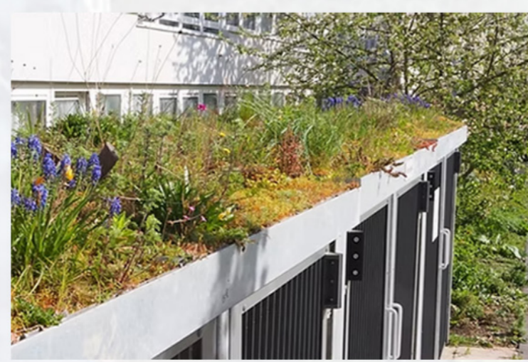
Green roof on cycle store
