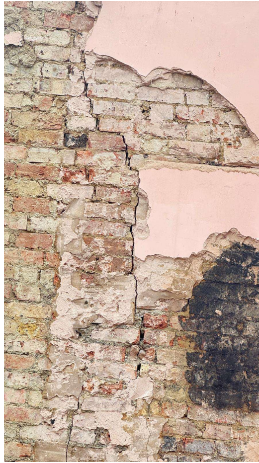
(b) Close-up of category 3 cracks of wall above mentioned in Pic (a)
