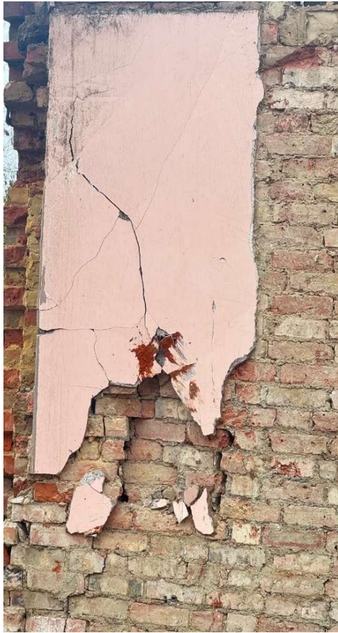
(b) Close-up of category 3 cracks of wall above mentioned in Pic (a)
