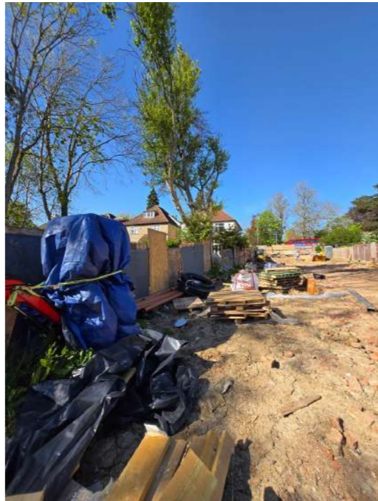
Site photo 2 facing north (T1 centre)
