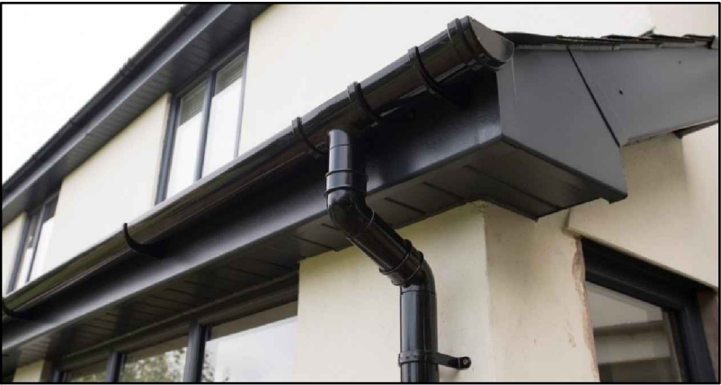
GUTTER & FASCIA COLOUR : BLACK FINISH : UPVC LOCATION : BUILDING GUTTER LEVEL
