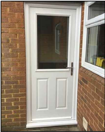
FRONT DOOR COLOUR : WHITE FINISH : HALF GLAZED COMPOSITE LOCATION : TO FRONT WALL
