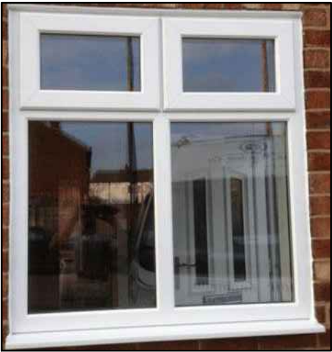
WINDOWS COLOUR : WHITE Aluminium frame WINDOWS FINISH : POWDER COATED ALUMINIUM LOCATION : TO EXTERNAL WALL
