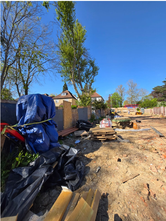
Site photo 2 facing north (T1 centre)
