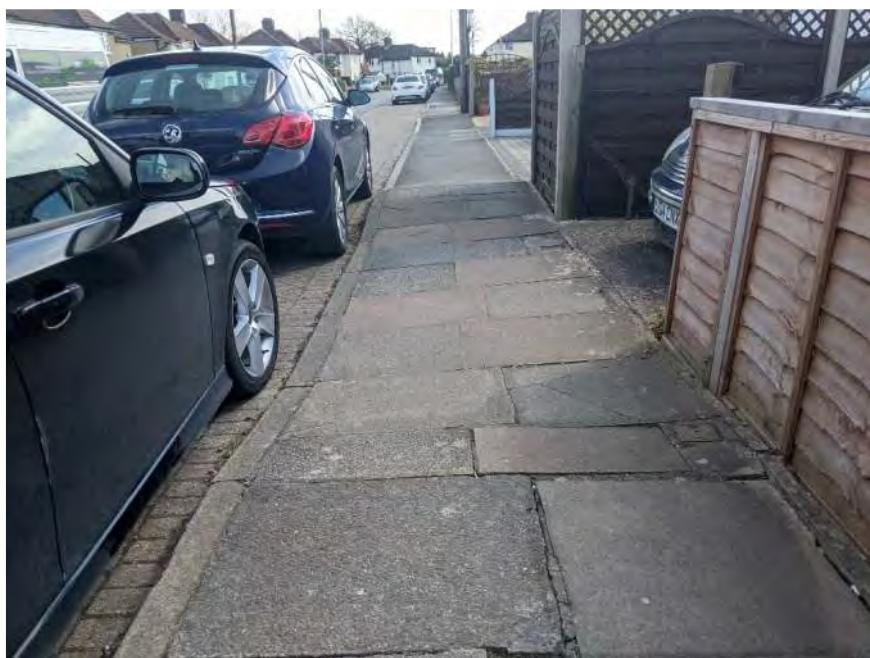
**Figure 5.8: Irregular paving and level at driveway access**
