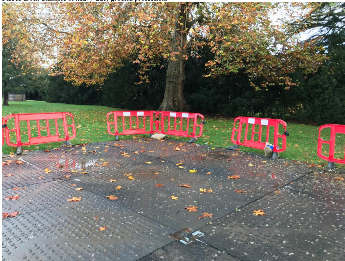
Photo 2. An example of heavy-duty ground protection.
