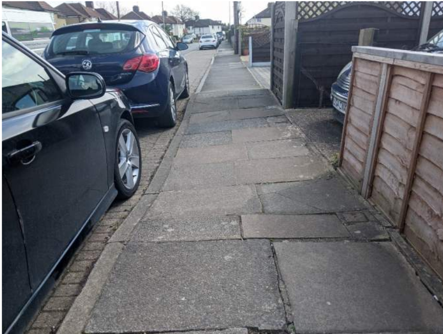
Figure 5.8: Irregular paving and level at driveway access
