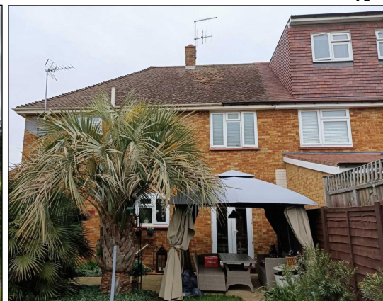
View of rear elevation
