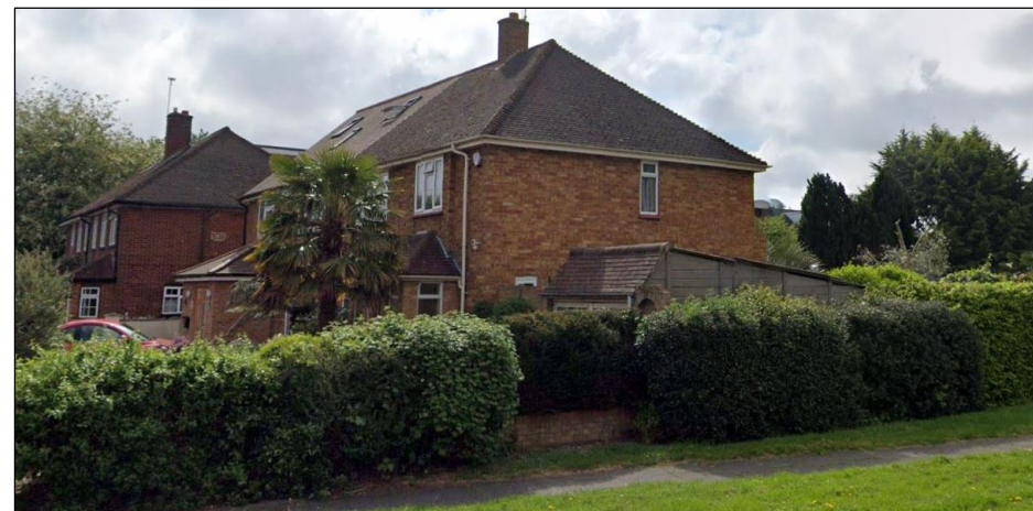
View of the house from the Maygoods Close and Maygoods Lane junction
