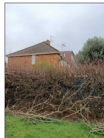
View of side elevation from Maygoods Close
