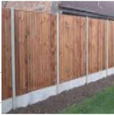
1.8m close boarded timber fence on concrete posts and concrete gravel boards with 30cm trellis above.
