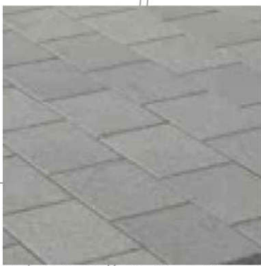
Marshalls Celestia Smooth Ground Flag Paving - Nebula 600x300x50. Laid to manufacturers specification.
