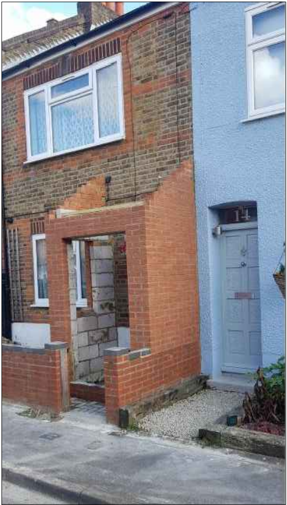
Partly erected front porch (Veiw 2)
