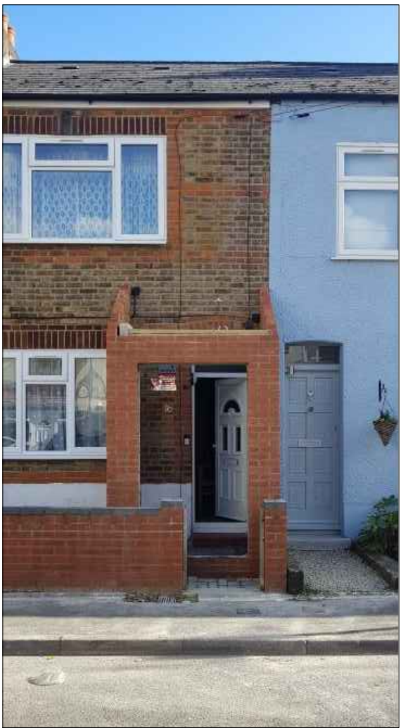
Partly erected front porch (Veiw 1)
