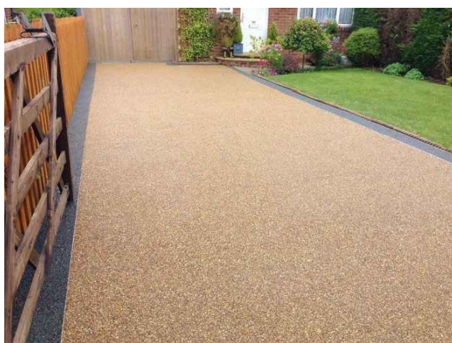
RESIN BOUND PERMEABLE PAVING BUFF COLORED RESIN BOUND PATHWAY https://www.westlondonsurfacing.co.uk/resin-bound/ Resin bound paving fixes together small stones with high-tech resin to form a firm, attractive surface. It creates many small gaps that allow water to drain through into the ground.
