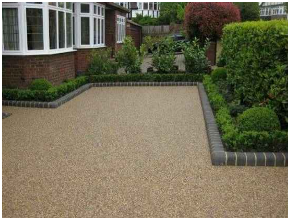
RESIN BOUND PERMEABLE PAVING BUFF COLORED RESIN BOUND PATHWAY https://www.westlondonsurfacing.co.uk/resin-bound/ Resin bound paving fixes together small stones with high-tech resin to form a firm, attractive surface. It creates many small gaps that allow water to drain through into the ground.
