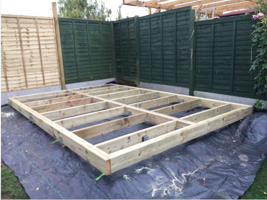
Base frame installed
