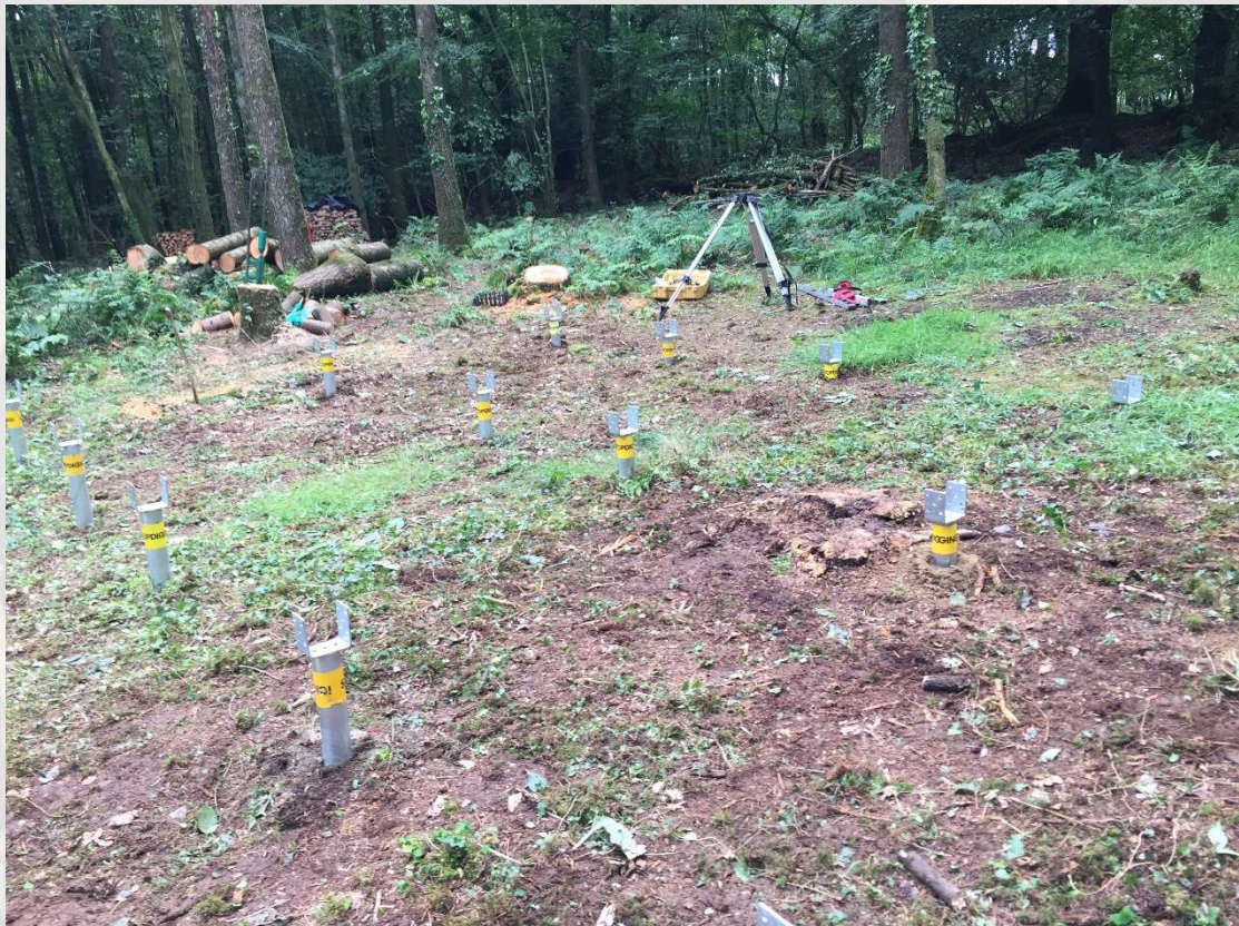
Screws installed ready for base frame
