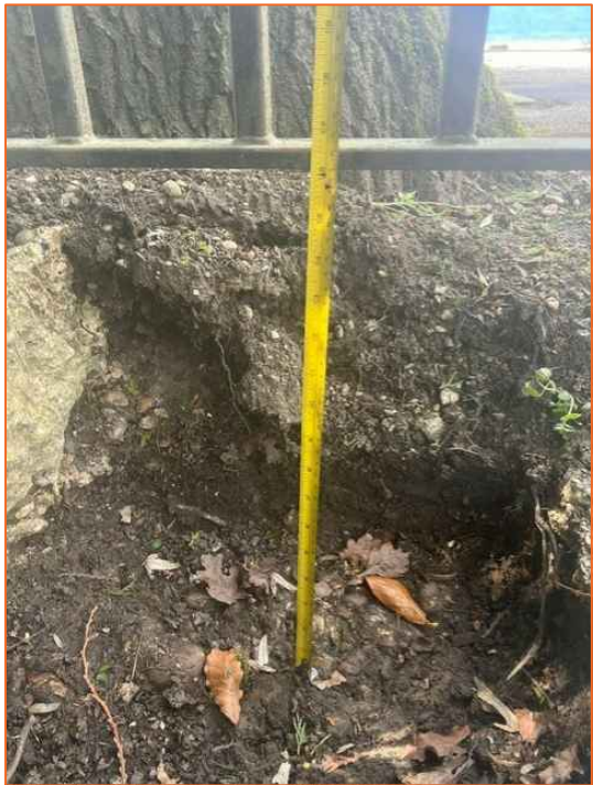
TRIAL HOLE EXCAVATED AT 600mm DEPTH SHOWING NO PENETRATION TO TREE ROOTS.
