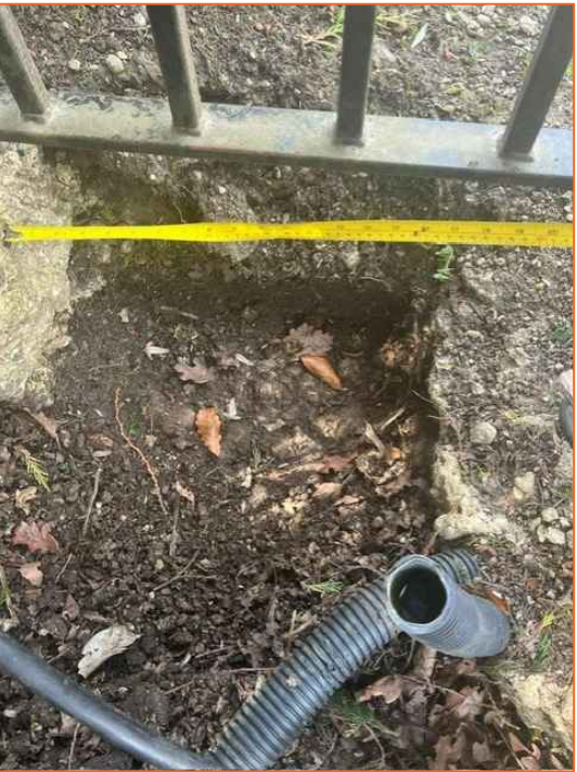
TRIAL HOLE EXCAVATED AT 500mm WIDE
