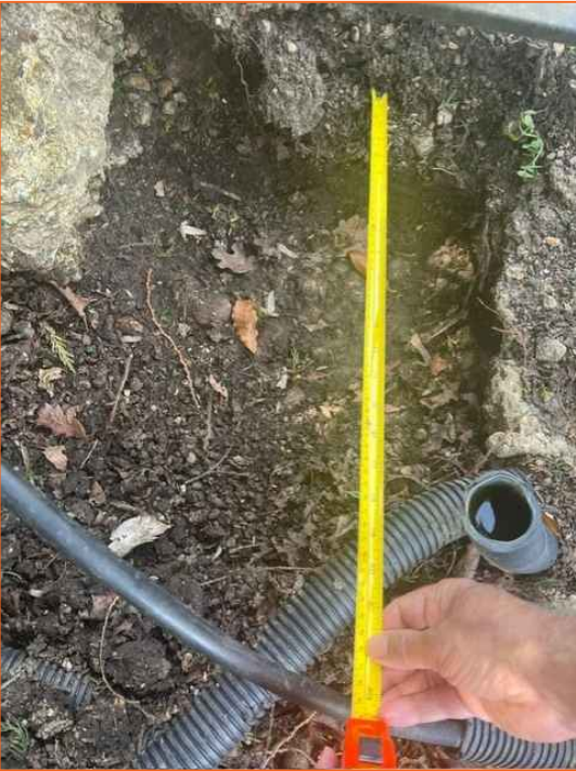
TRIAL HOLE EXCAVATED AT 650mm FROM EXISTING RAILINGS
