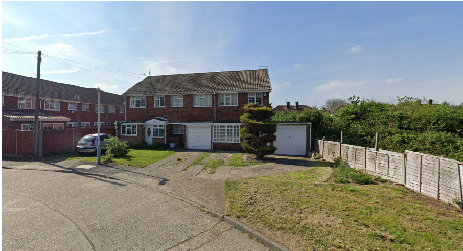
View of Front 50 Manor Lane
