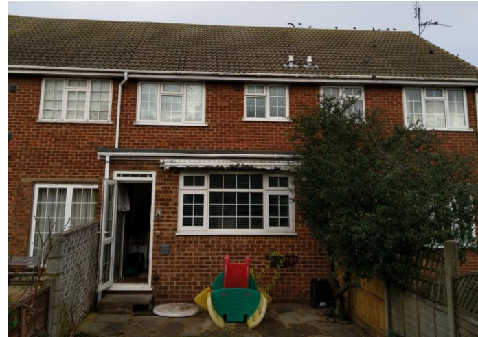
View of Rear of 50 Manor Lane
