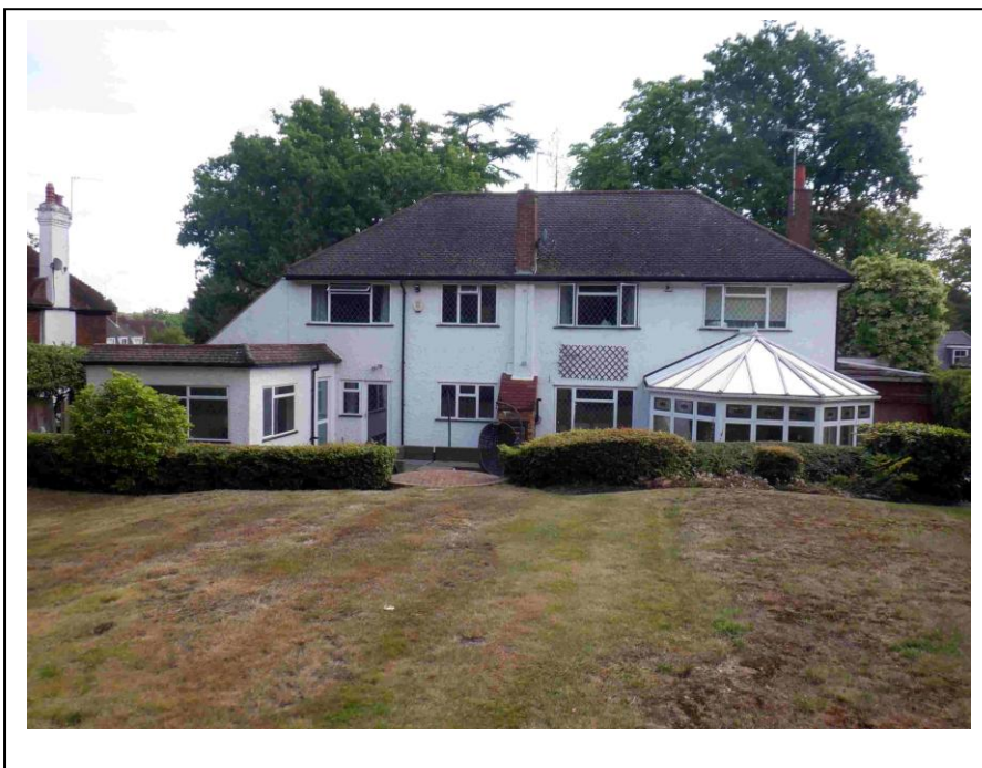
View of the rear elevation
