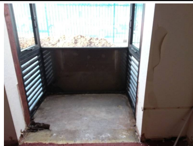
Former Work Area
