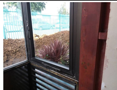
Former Work Area
