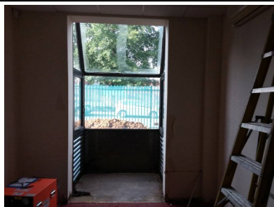
Former Work Area
