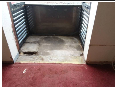
Former Work Area
