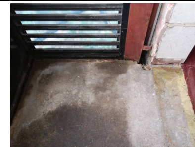
Former Work Area
