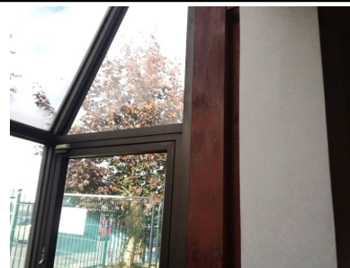
Former Work Area
