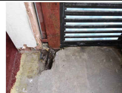
Former Work Area
