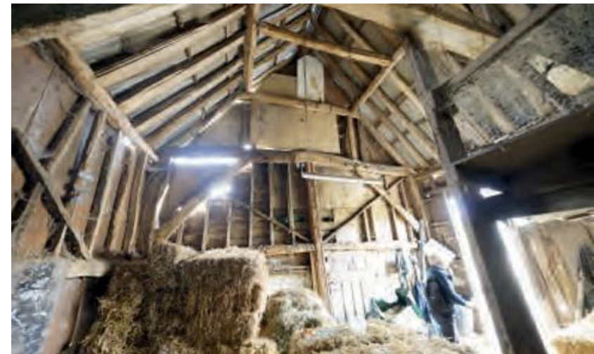
Internal view of retained barn
