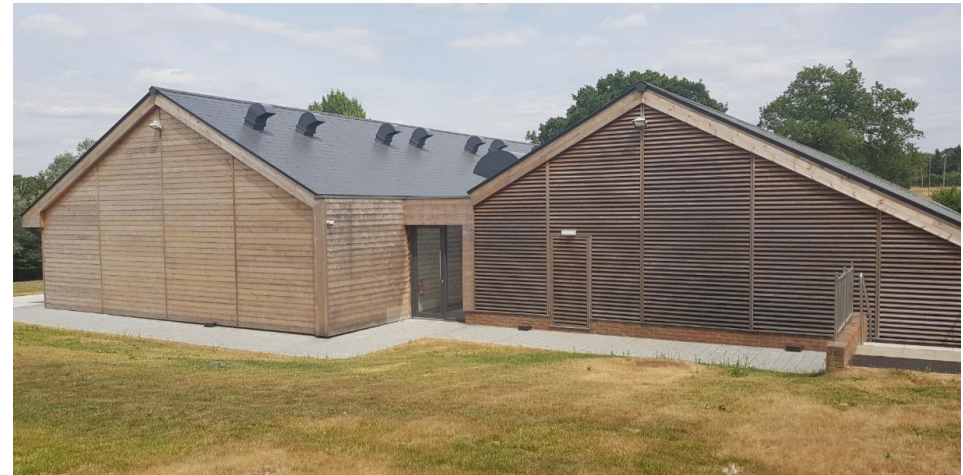
View of the western gables of the function space / kitchen building
