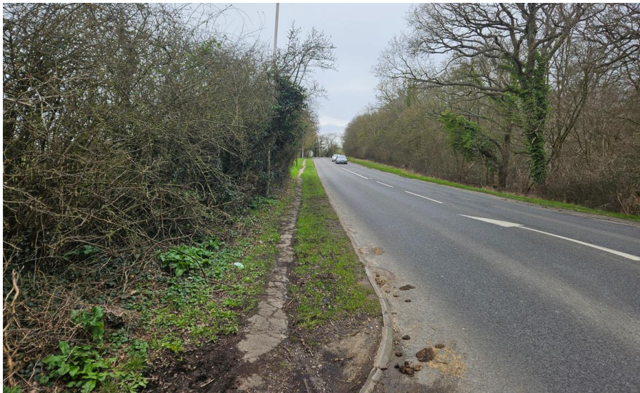
View from the site access looking north
