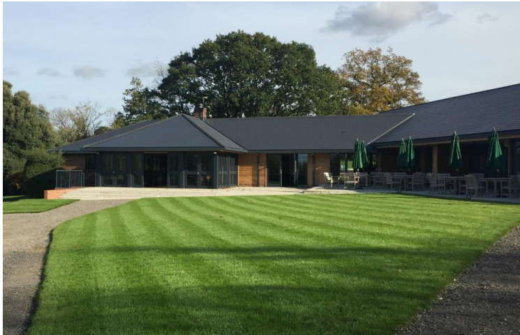
View toward the reception building and function space
