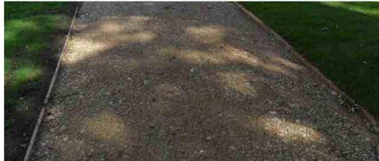
Gravel finish to sit flush with the adjacent field and to have very thin edging strips. The path will not have any fencing either side to ensure a discreet presence in the landscape
