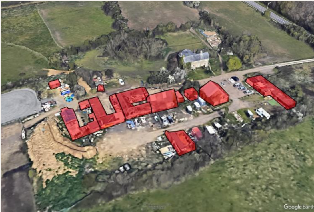
Figure 7 – Extent of the Demolition Proposal (Pre-Demolition Audit by Velocity)
