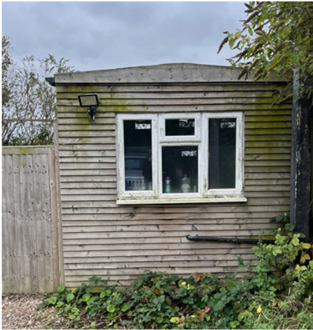
Figure 4-3 Timber Cladding - Staff Rest Room
