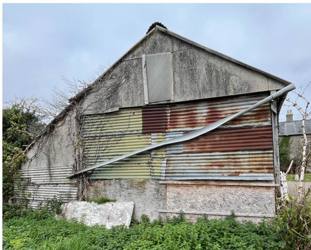
Figure 2-4 Repaired Façade – Large Stable
