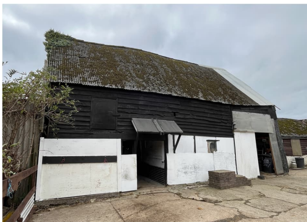
Figure 2-3 Large Stable Frontage - Concrete Blocks
