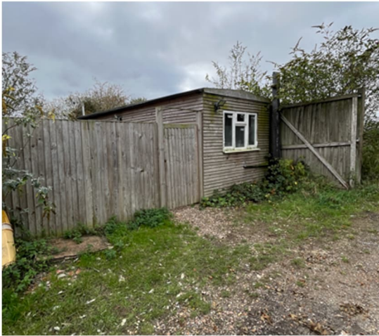
Figure 2-12 Staff Rest Room
