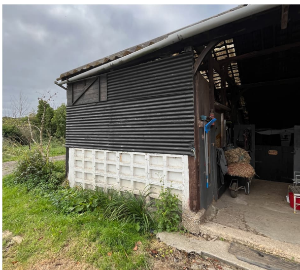
Figure 2-3 Large Stable Frontage - Concrete Blocks
