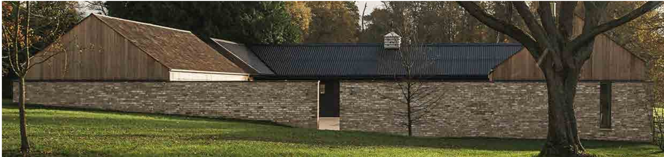
Downland Barns, Mclean Quinlan Architects : Reclaimed brick 'garden wall' with pitched volumes above in a different material helps ground and unify the building whilst also providing the necessary articulation. We have adopted this approach in the design of our South Elevation which is effectively the 'rear' of the building.
