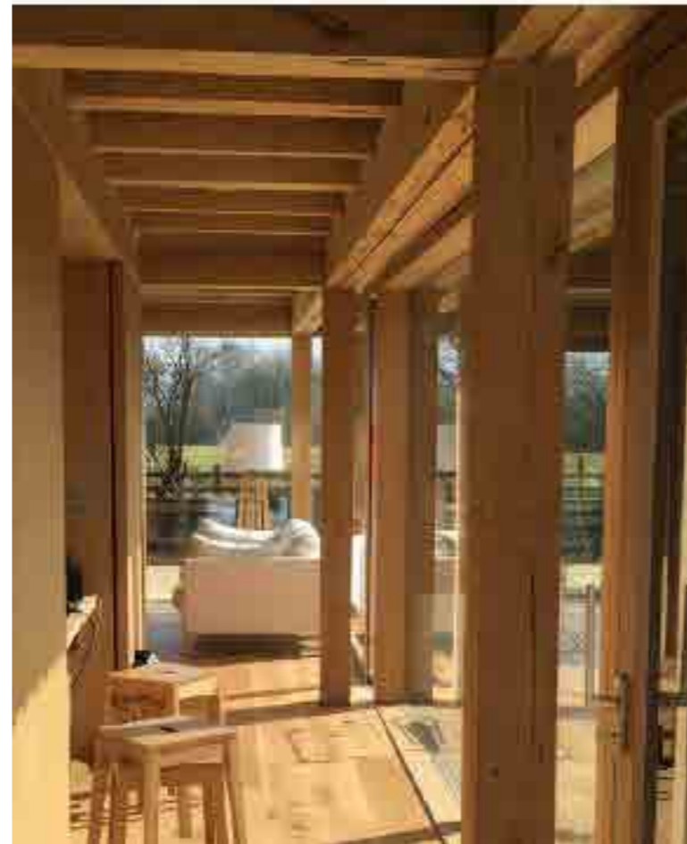
Contemporary precedent image of a solid oak-framed structure expressed internally. This project is a previous work by the Structural engineer for the workshop project (MHA Associates).
