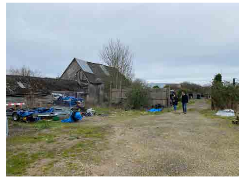
View from South West showing existing areas of hard-standing. West and South elevations of Principle Heritage Barn (Barn A) visible in centre of image.
