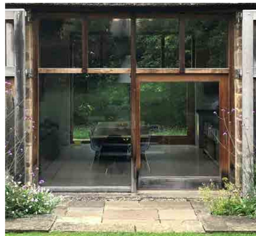
Chestnut Farm, Rutland: Generously proportioned glazing apertures to maximise light whilst incorporating traditional timber framing and glazing bars
