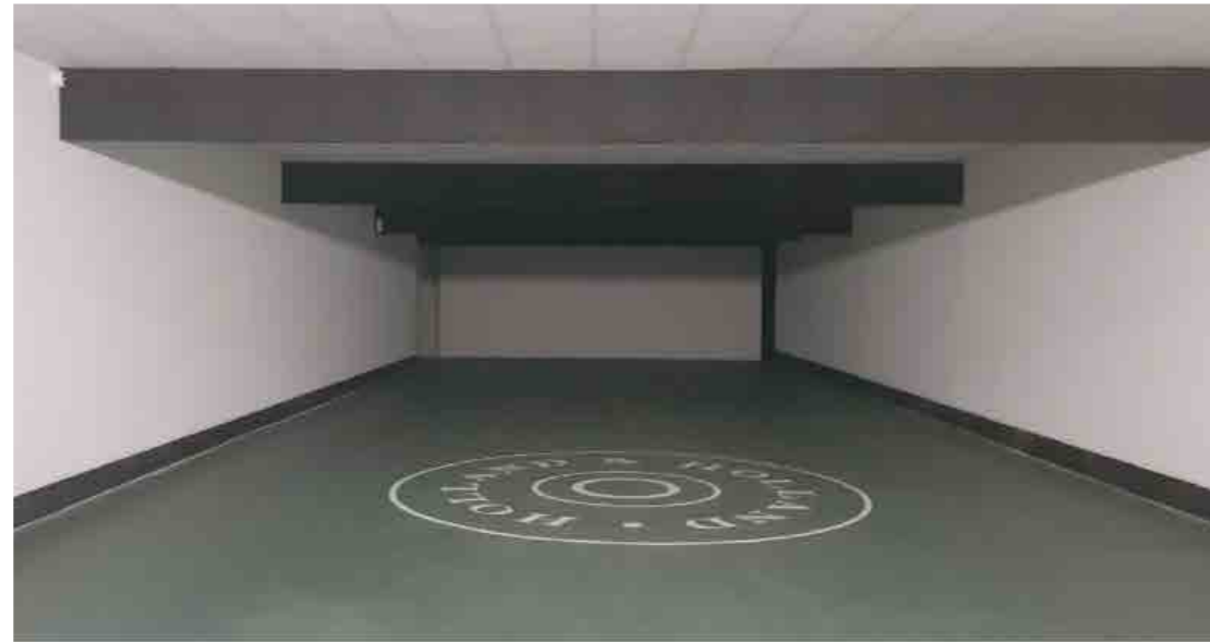
Underground Shooting Range
