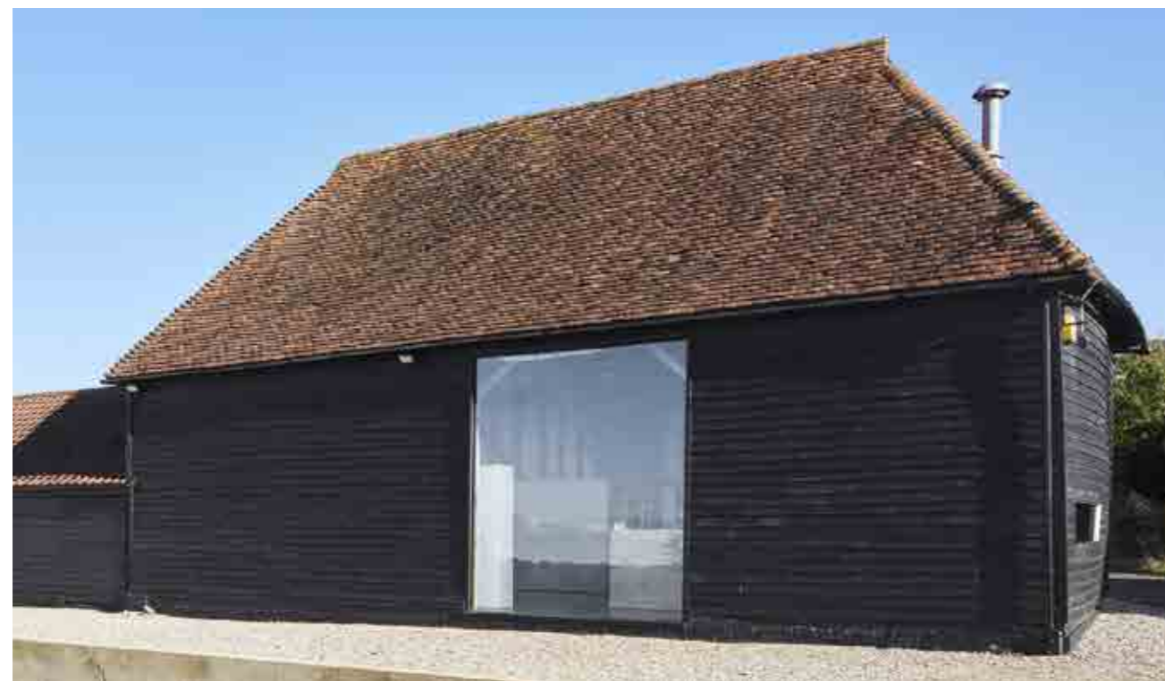
Tilty Barn, Essex : Traditional black shiplap boarding and red keymer clay tiles. Large glazed apertures to maximise light into the double-height interior space of the barn also serve in their proportion to give the barn a sense of hierarchy within the overall facade composition.
