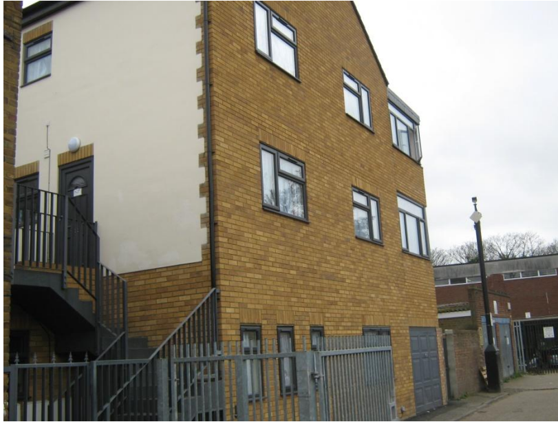
Figure 6 -View from Service Road
