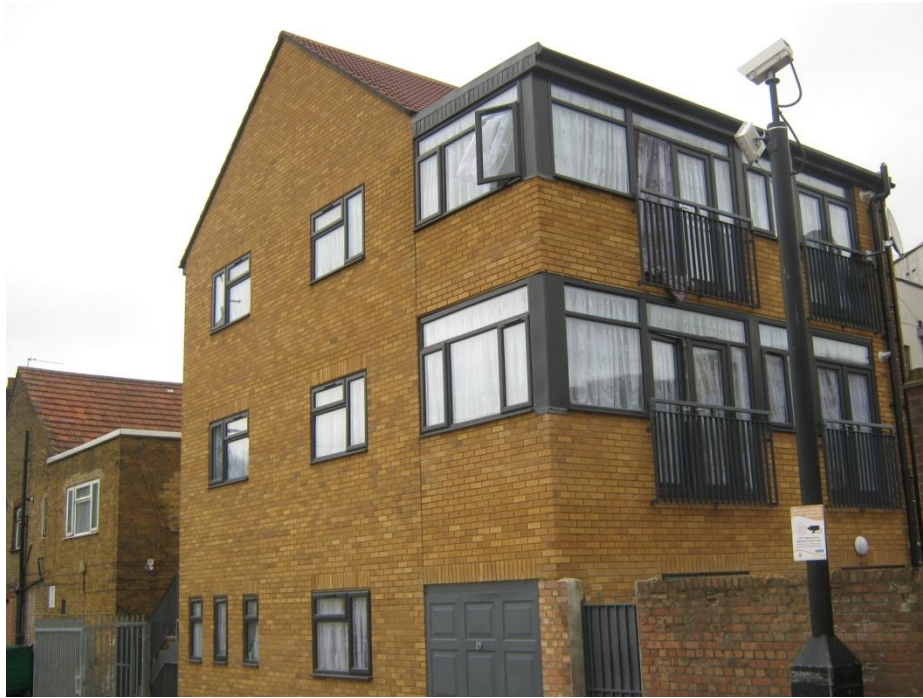
Figure 5 - Rear Extension as built
