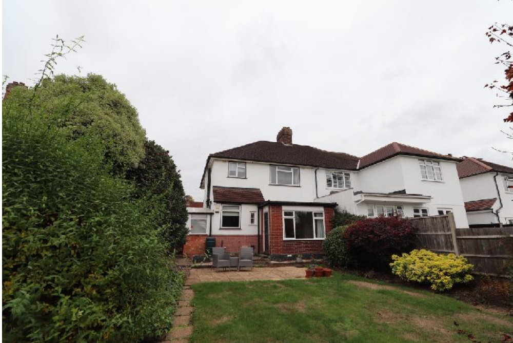
Rear photo showing the adjoining property number 9 which has benefited from a two storey rear extension 3.6 m deep.
