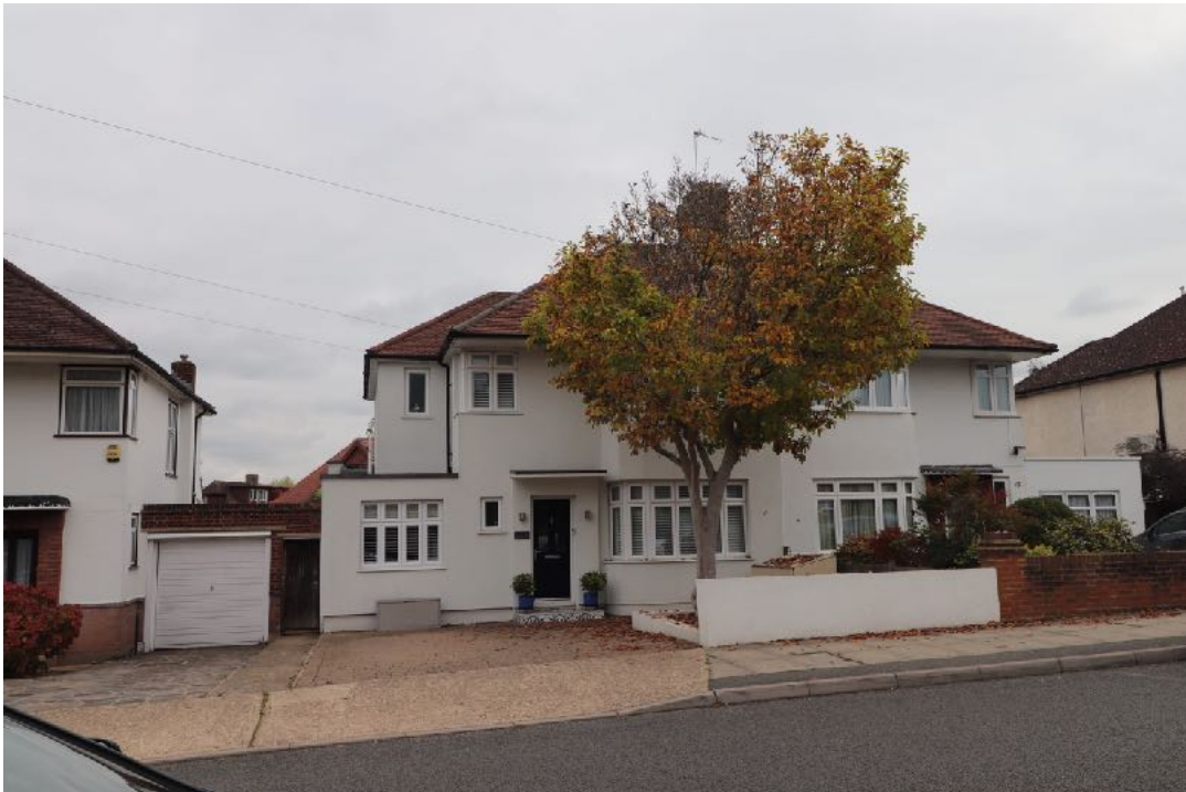
Example of similar extension at number 13 Manor Way
