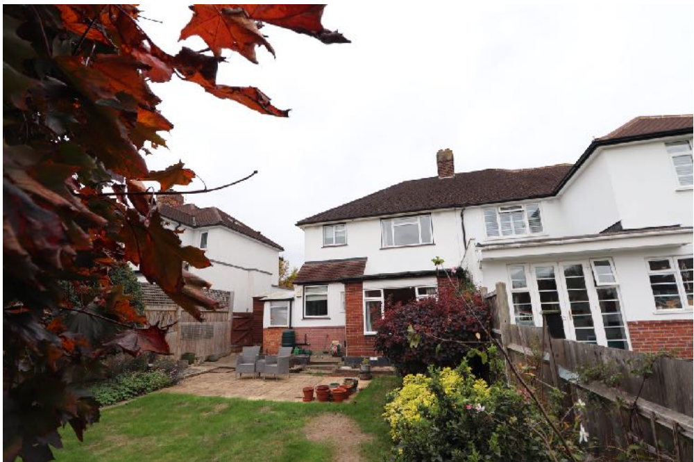
Rear photo showing the adjoining property number 13 which has also benefited from a two storey rear extension.
