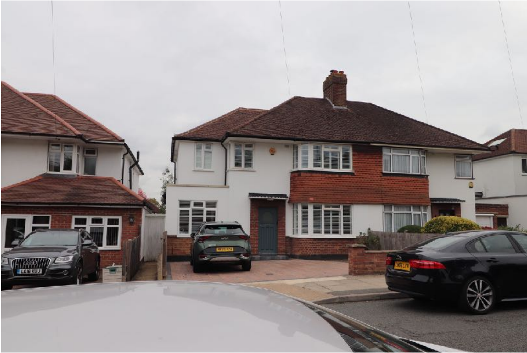
Example of similar extension at number 9 Manor Way
