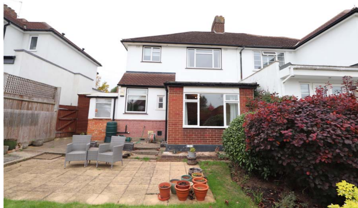
Rear view showing 11 Manor Way and rear extension to 13 Manor Way
