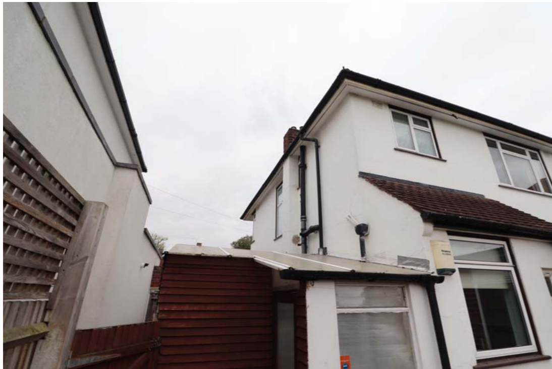
Rear view of garage and lean too
