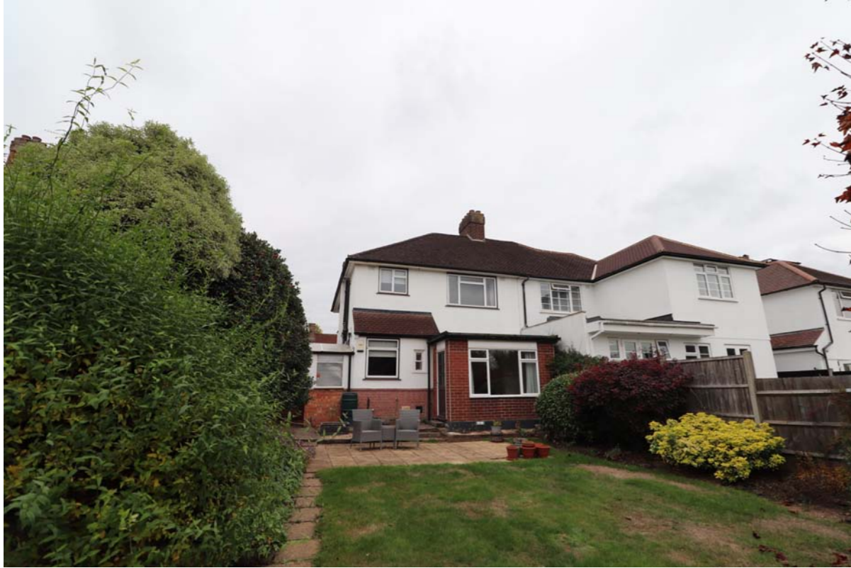
Rear view showing 11 Manor Way and rear extension to 9 Manor Way
