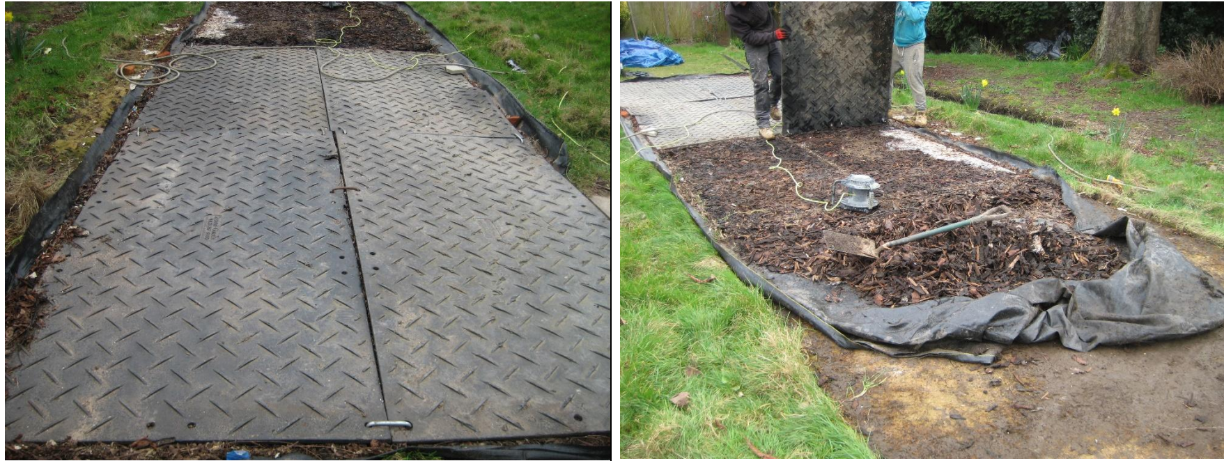
Fig 10 – Temporary ground protection is an effective way of allowing access through the RPA of retained trees. It must be installed prior to any on site activity and maintained for the duration of all works to be effective. Above left Tamla Trees project ground protection in place and above right being removed following the completion of site works. (Note: depending on the length of time it is in place it will adversely affect underlying grass ground cover which will need reseeded/ turfed accordingly)
