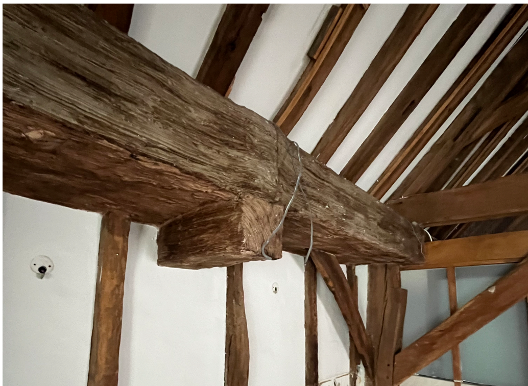
One of the artificial (fibreglass) beams on the first floor, above the aisle
