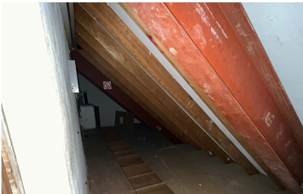
Steel beam in use as a principal rafter
