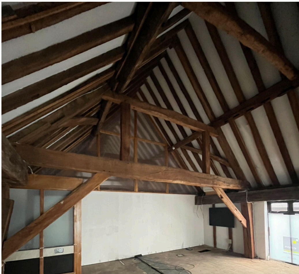
First floor interior, showing the floor inserted in 1977 and one of the original queen post trusses. The partition behind was formed in 2012
