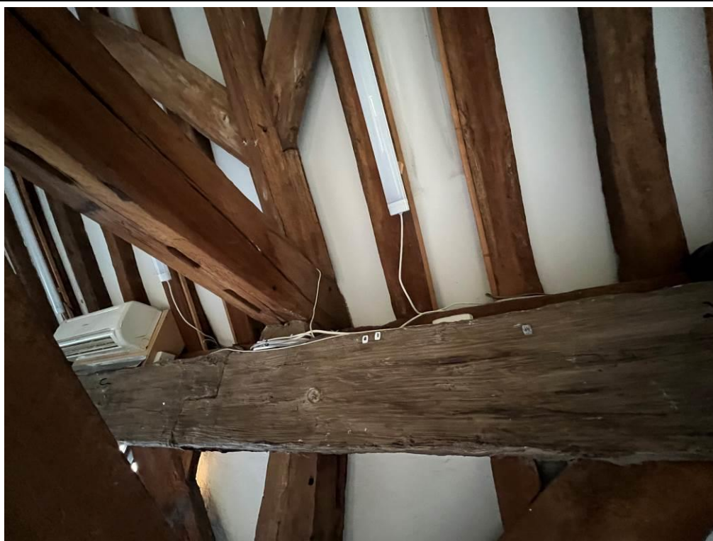
Figure 3 – Cheap surface mounted light fittings fixed to rafters
