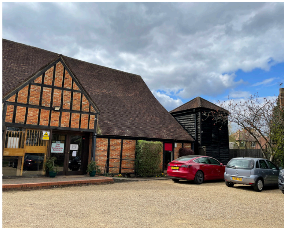
The Barn House / Field End Barn as viewed by Car Park
