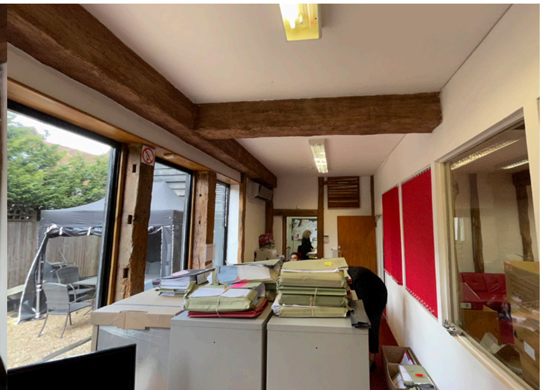
Main barn ground floor interior at point of proposed extension
