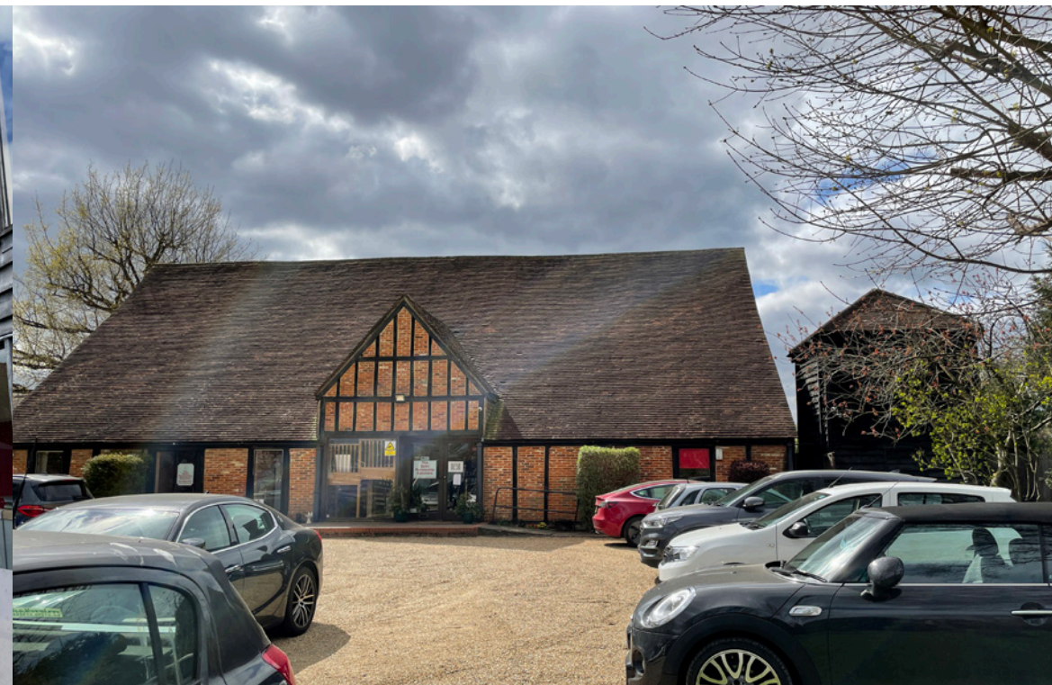
The Barn House / Field End Barn as viewed by Car Park
