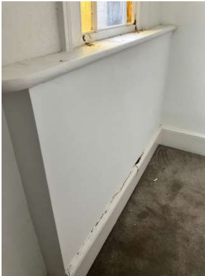
Photo 12 Wall below stair window showing damp to plaster and skirting
