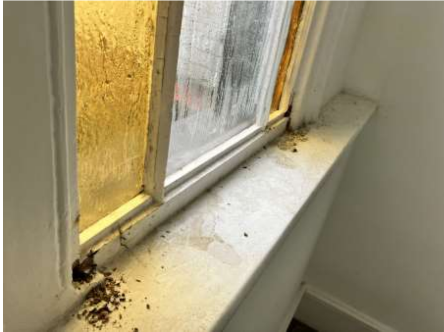
Photo 11 Stair window showing rot to cill and jambs and water on window board which drips onto wall below
