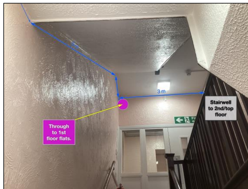
Plate 4: Indicative pipe route of internal gas riser pipework for Design Option 2.
