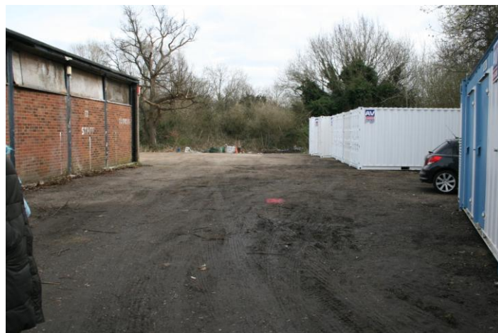
View of the site, looking east, in 2017, after the Council contractors had moved in
