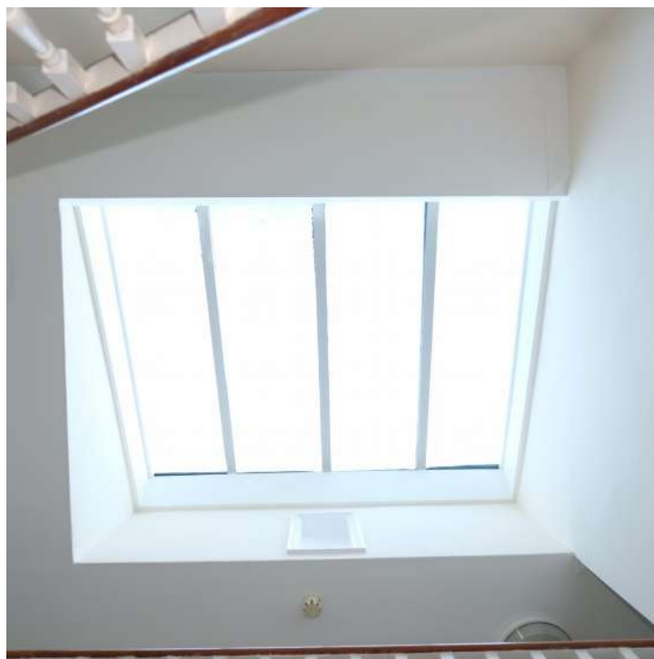
Plate 7 - Rooflight in room C, facing west from room J
