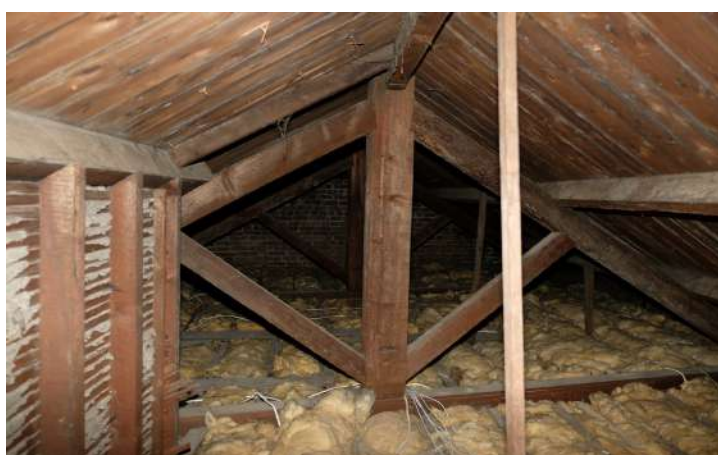
Plate 9 - Attic, facing west
