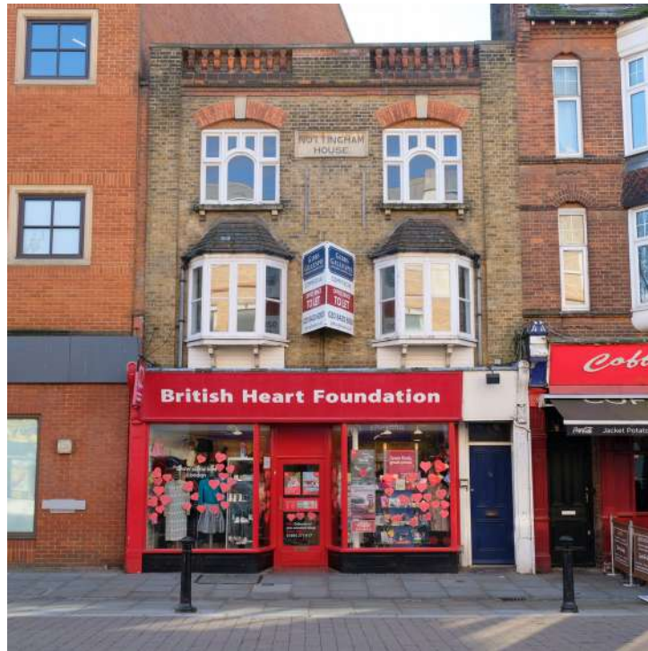
Plate 1 - High Street Façade
