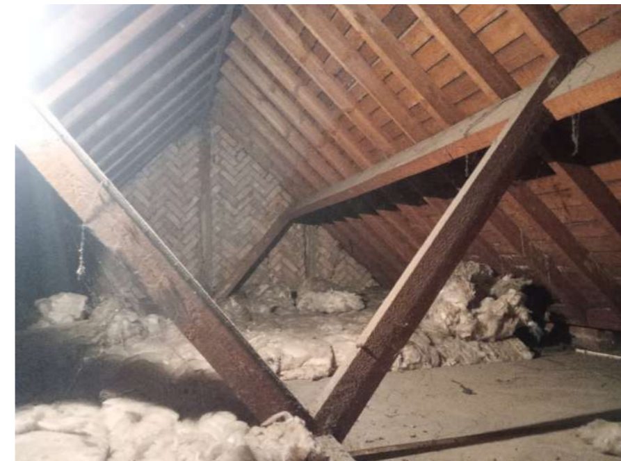
View inside loft space
