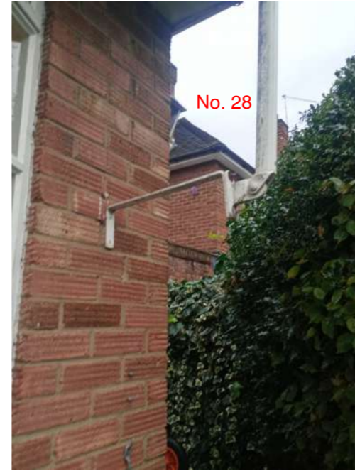
View from rear bay to No.28 boundary
