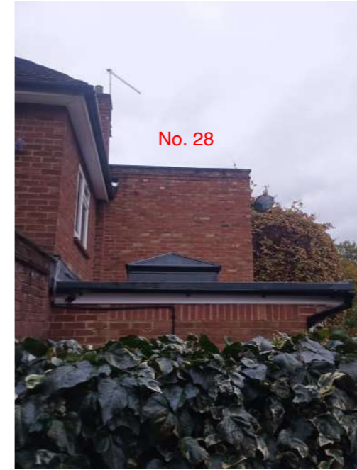
View from side to No.28 boundary
