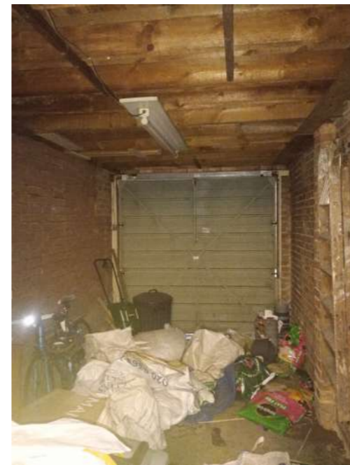
View inside garage to front
