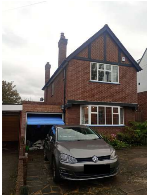
View from front drive
