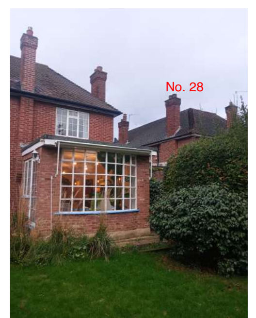
View from rear garden to No. 28
