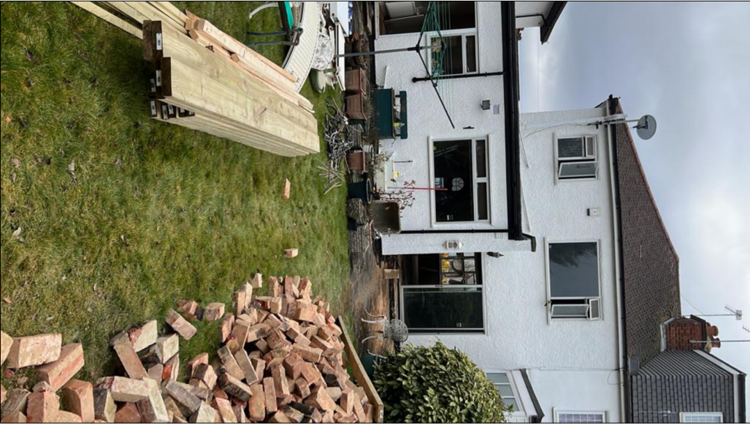
Pre-Existing rear view
