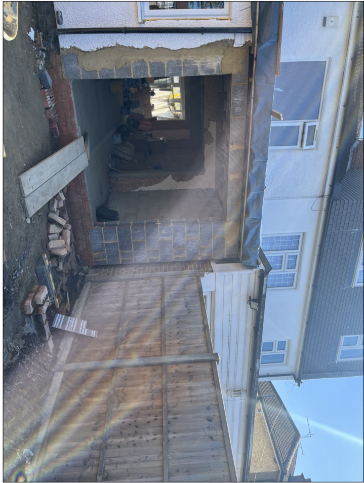
Existing rear extension
