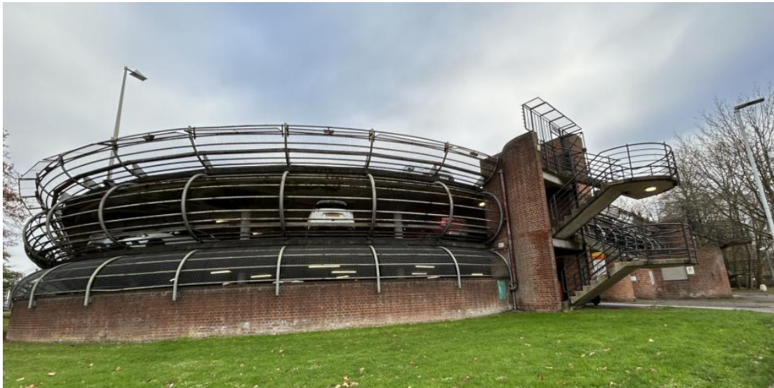
Fig 1. Existing Civic Centre Car Park, Uxbridge
