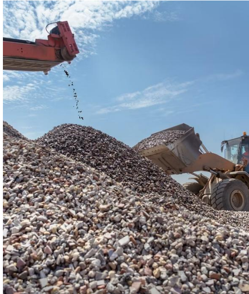
Fig 3: Illustration of reinforced concrete waste crushed to aggregates on site
