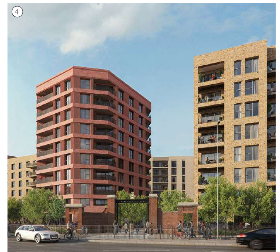
↑ St Andrews Park Development - 1300 new homes, 3-10 storeys
