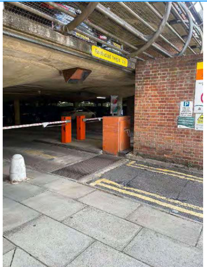
Carpark entrance from Cricket Field Road
