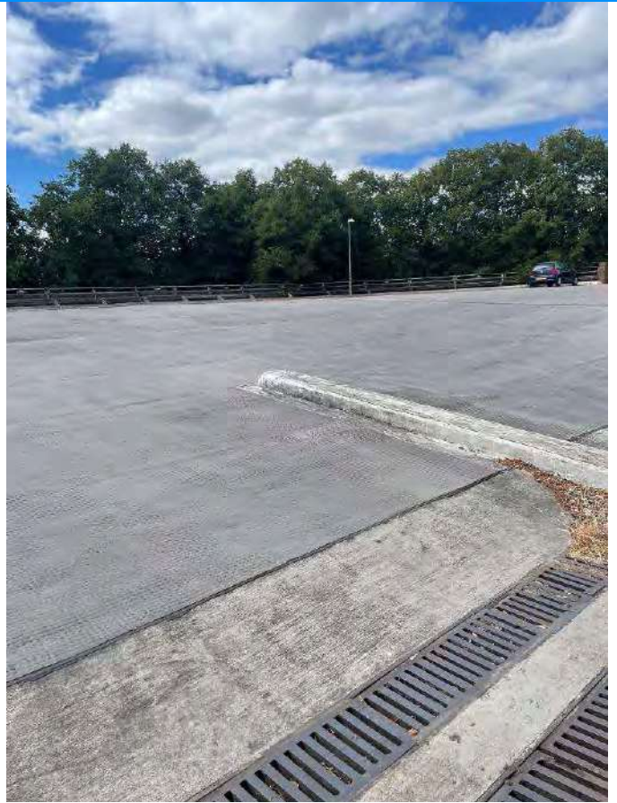
Drainage on carpark roof level
