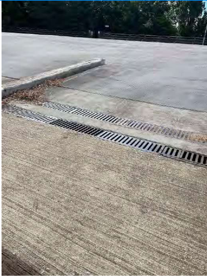
Drainage on carpark roof level
