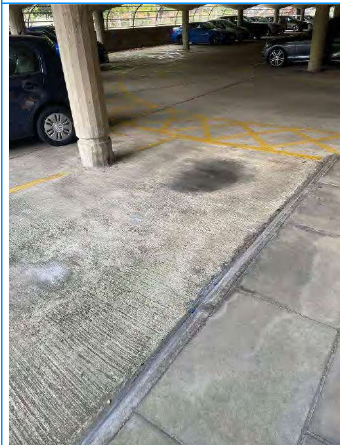
Ground floor level surfacing
