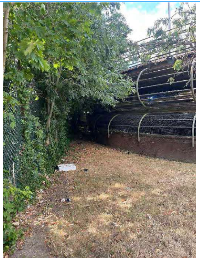
North-eastern corner of car park
