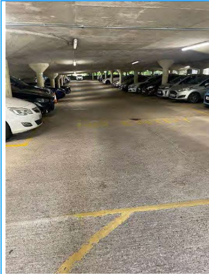
Overview inside multi-storey car park
