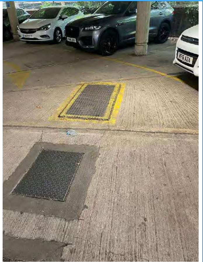
Utility inspections covers within the ground floor
