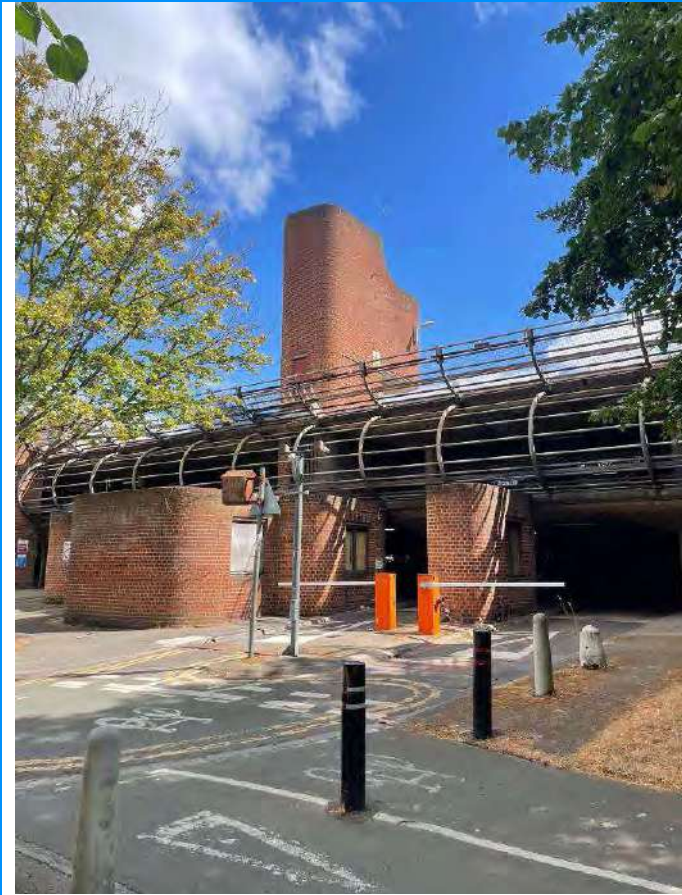
Carpark entrance from Cricket Field Road
