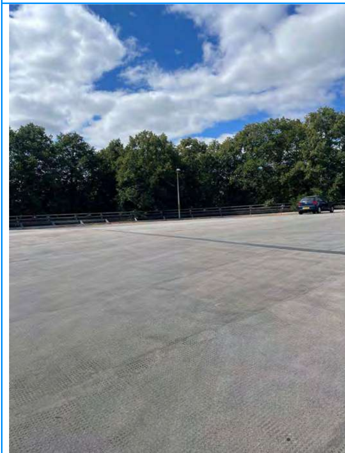
Overview of carpark roof level
