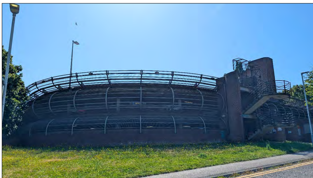
Photo. 1 View of the carpark from north-west, looking south-east
