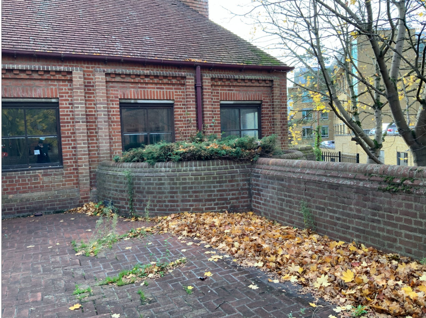
Existing Raised Podium
