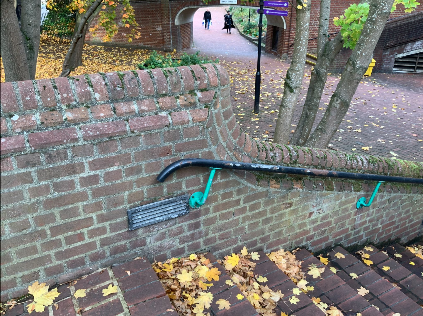
Existing Raised Podium
