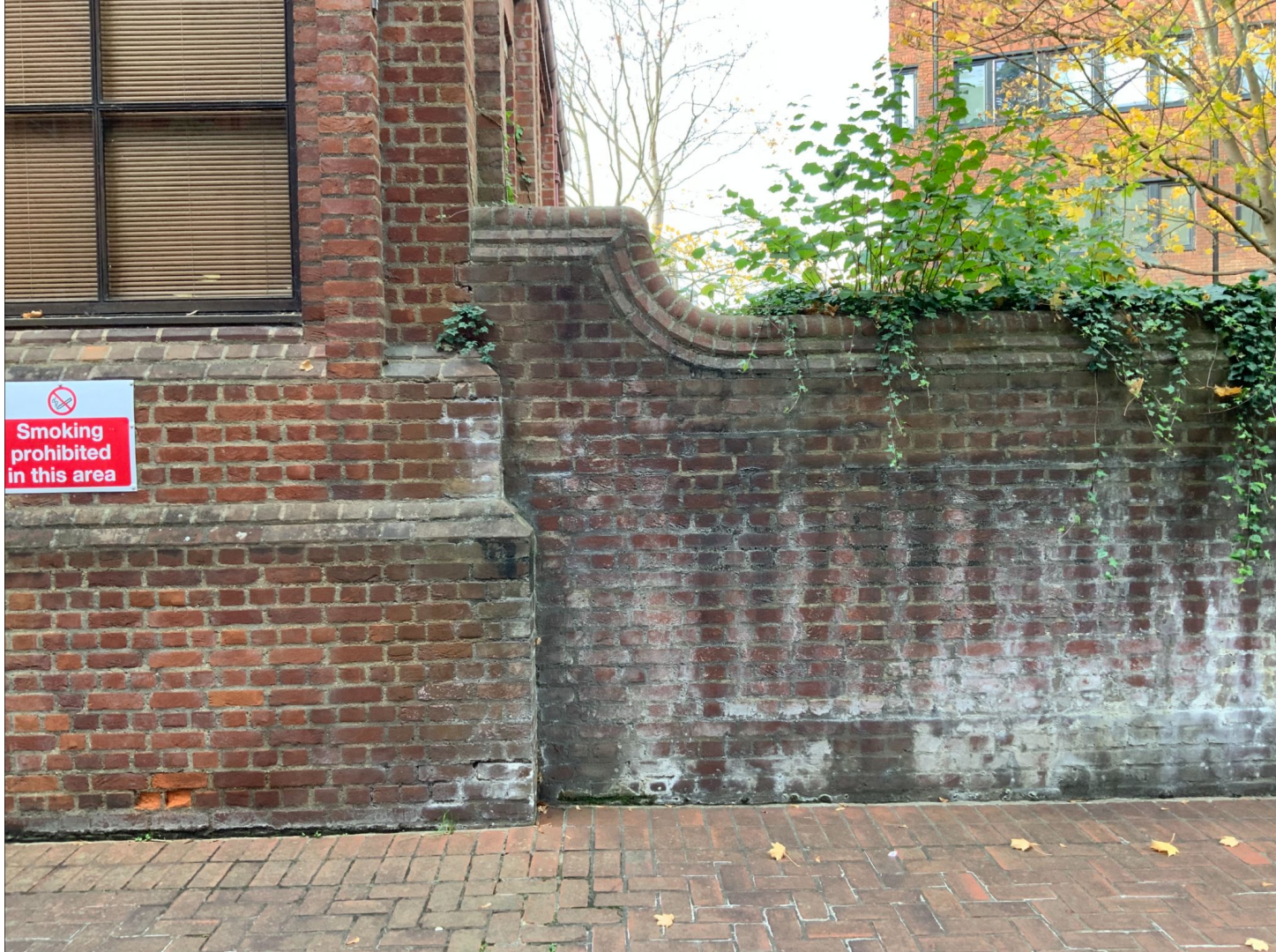
Existing Raised Podium
