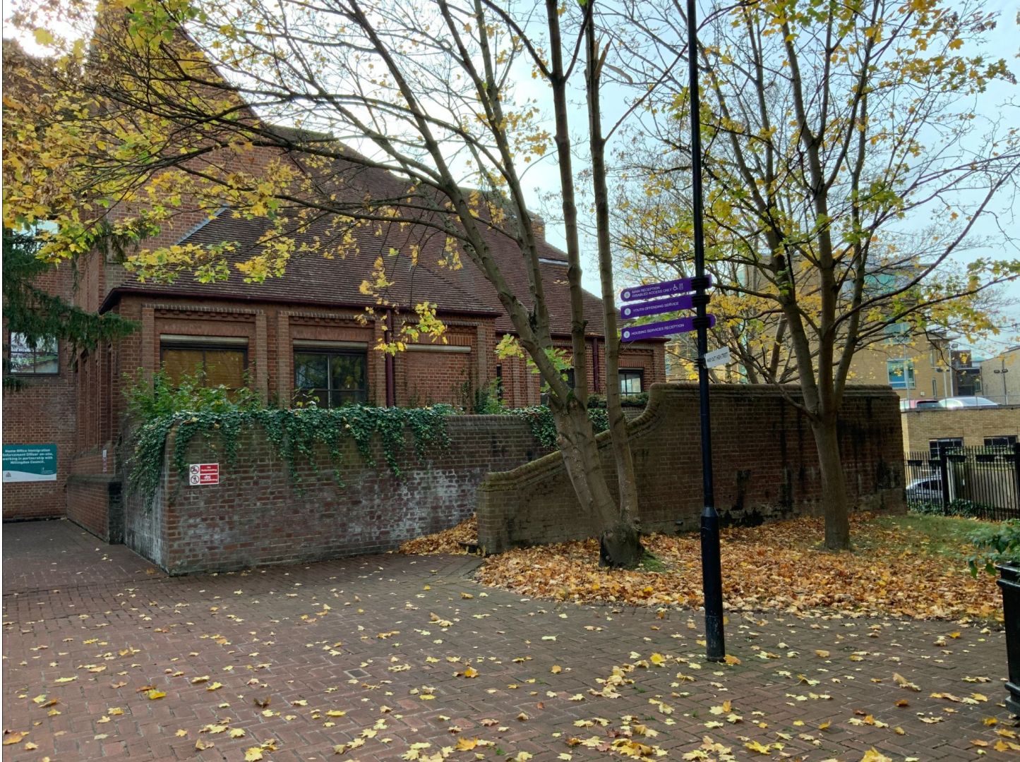
Existing Raised Podium
