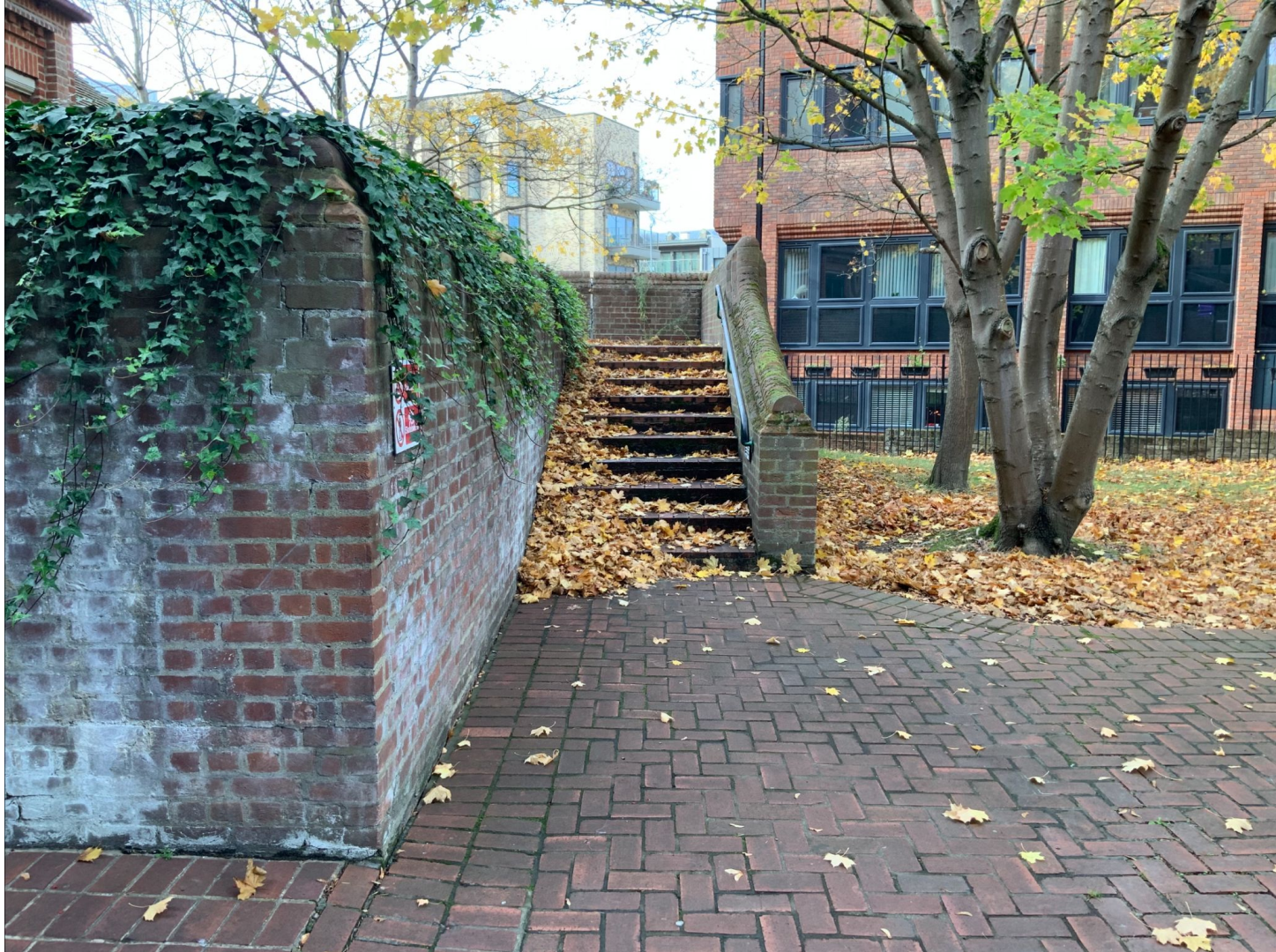
Existing Raised Podium
