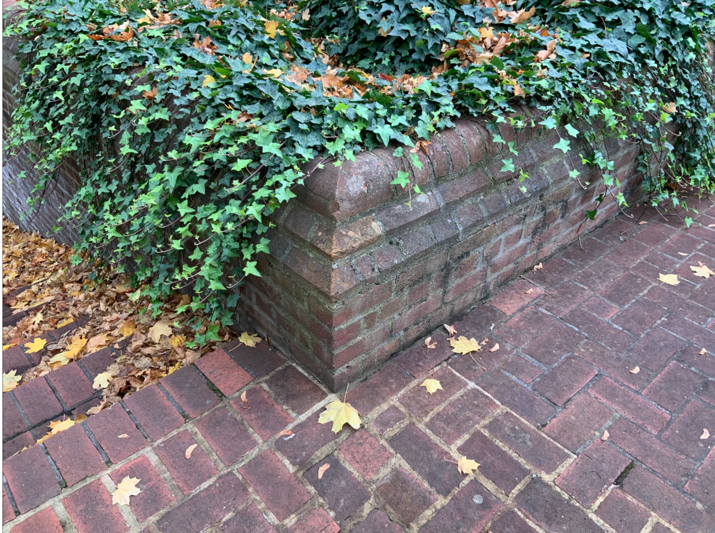
Existing Raised Podium
