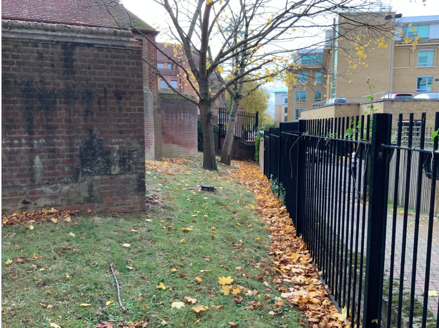
Existing Raised Podium
