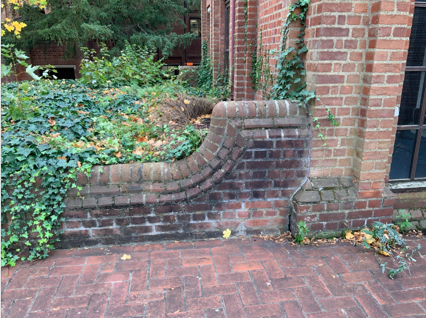
Existing Raised Podium
