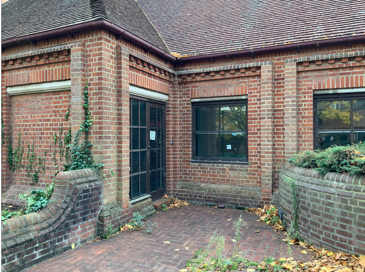
Existing Raised Podium
