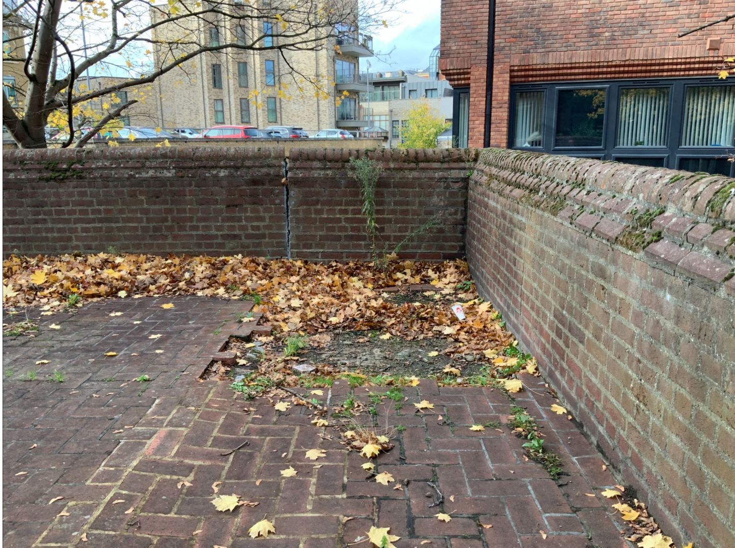
Existing Raised Podium
