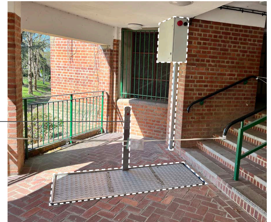
↑ Existing out-of-service pit-mounted platform stairlift
